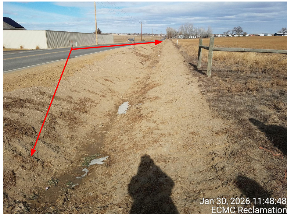
Photo 1. Photo taken from CR51 and the western portion of Parcel T089 at the surface owners driveway, facing North. Photo illustrates the Operator excavated soil from the roadside ditch.
