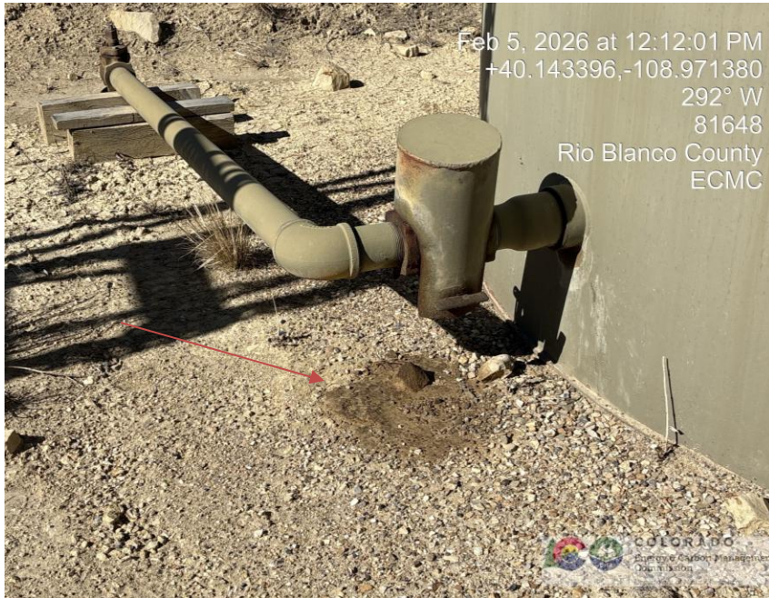
Photo # 1694 Staining on location near production tank unload line
