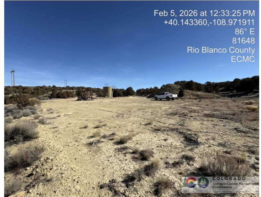
Photo # 1719 NW corner of location
