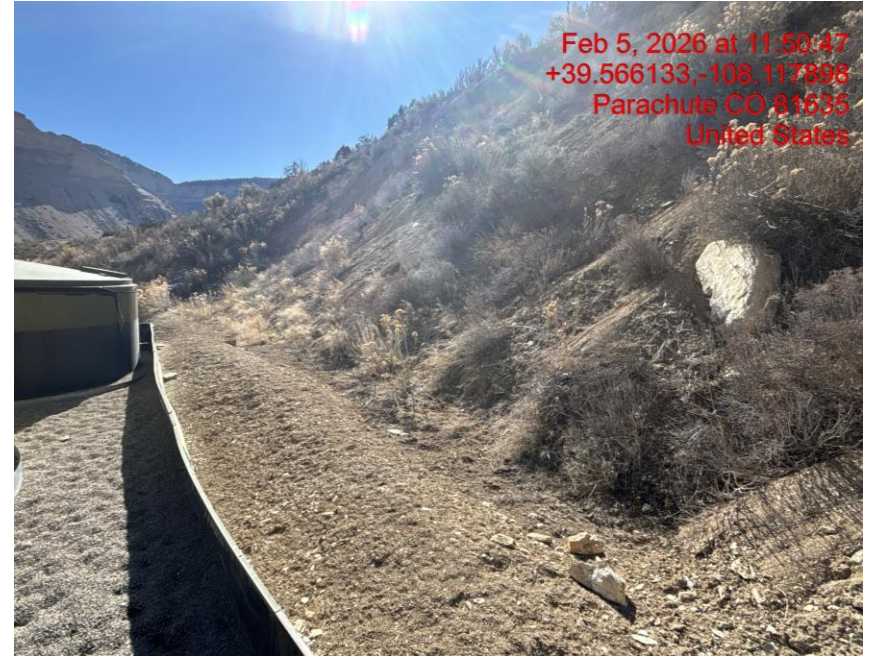
Cut Slope Erosion Encroaching into Secondary Containment – Photo #02641
