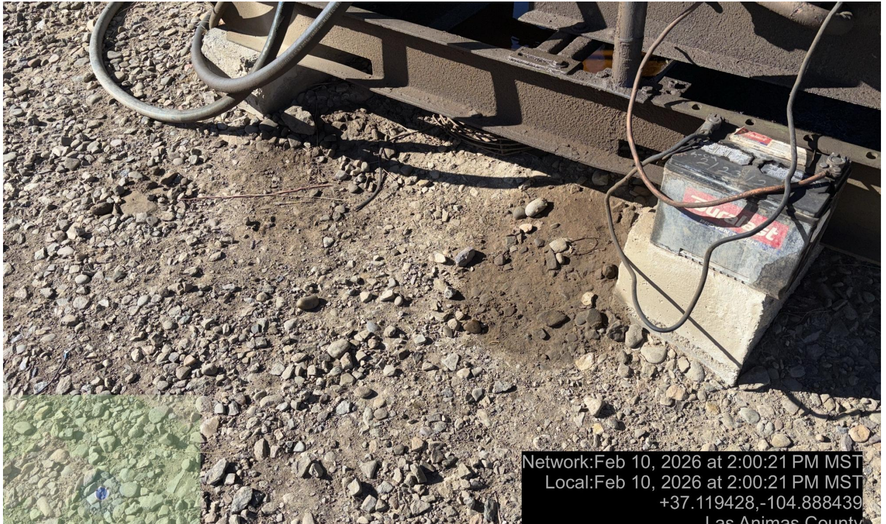
PHOTO 6: Area of impacted soil near prime mover engine skid. Conduct maintenance on equipment, cleanup stained material and review self inspection processes. COMPLY WITH RULE 1002,(2).D. ca date 2/23/2026.
