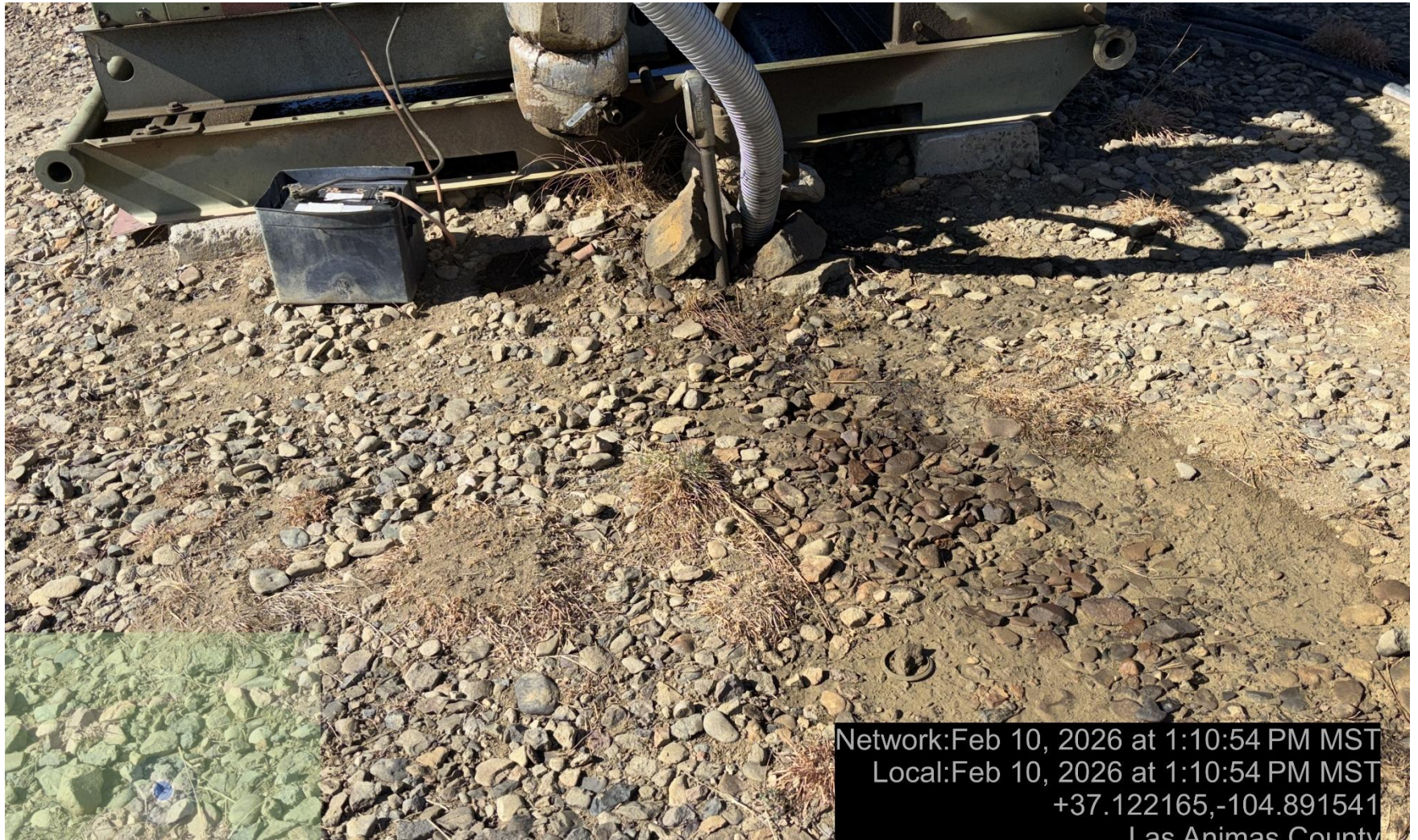
PHOTO 7: area of impacted soil near prime mover engine skid. Conduct maintenance on equipment, cleanup stained material and review self inspection processes. COMPLY WITH RULE 1002,(2).D. ca date 2/23/2026.
