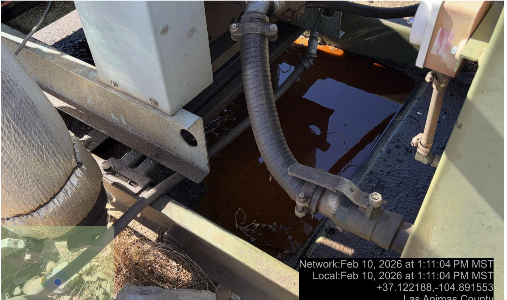
PHOTO 11: OILY WASTE IN PRIME MOVER ENGINE SKID WITHOUT WILDLIFE PROTECTION SCREENS OR COVERS. DRAIN OILY WASTE REPAIR ALL LEAKS AND REMOVE IMPACTED SOIL PER RULE 1002..(2).D & 1002.f.(2)B, Comply with general provisions of the oil and gas act for wildlife protection AND SB-181. IMMEDIATE ACTION IS REQUIRED. CA DATE 2/11/2026.
