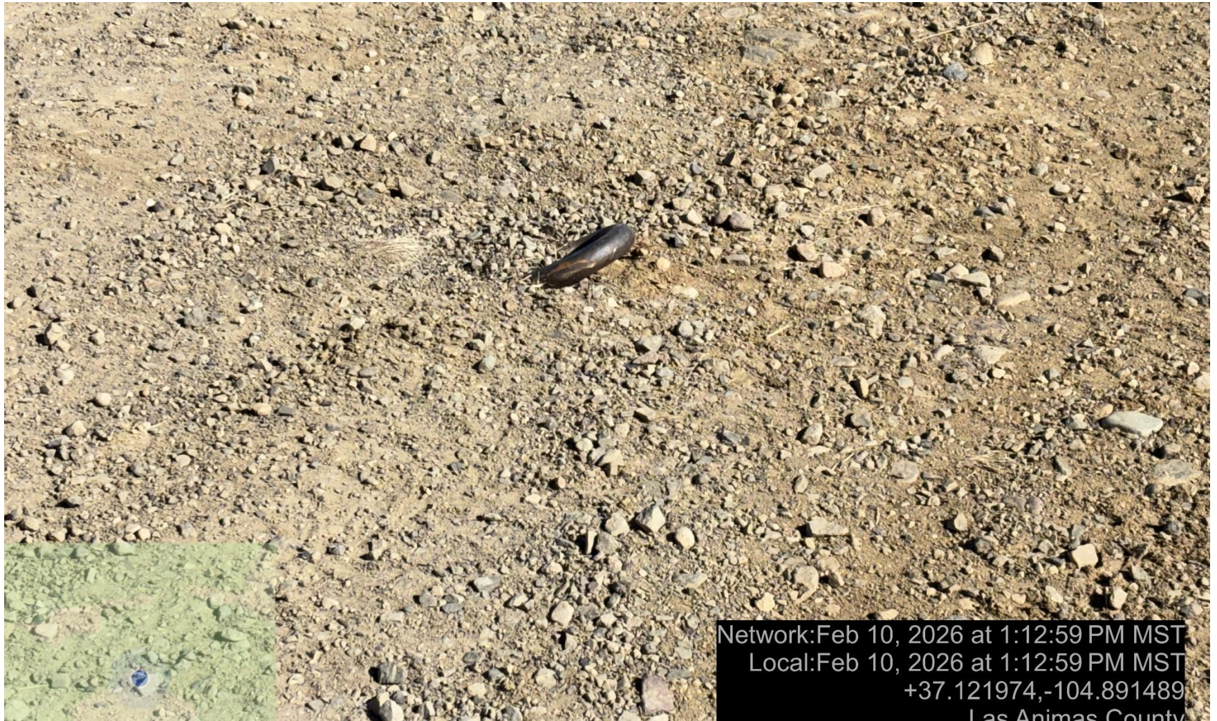
PHOTO 10: no guy line marker on southeast anchor. Install proper guy line markers per Rule 1003.a. ca date 2/23/2026.
