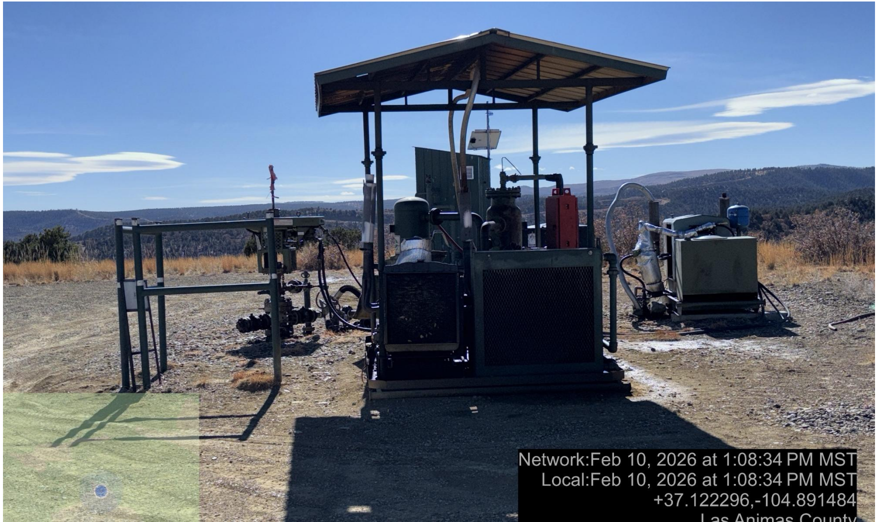
PHOTO 4: Vacuum pump observed on well without ECMC approval. Provide ECMC with documentation showing approval of use of vacuum pump. Ca date 2/23/2026.
