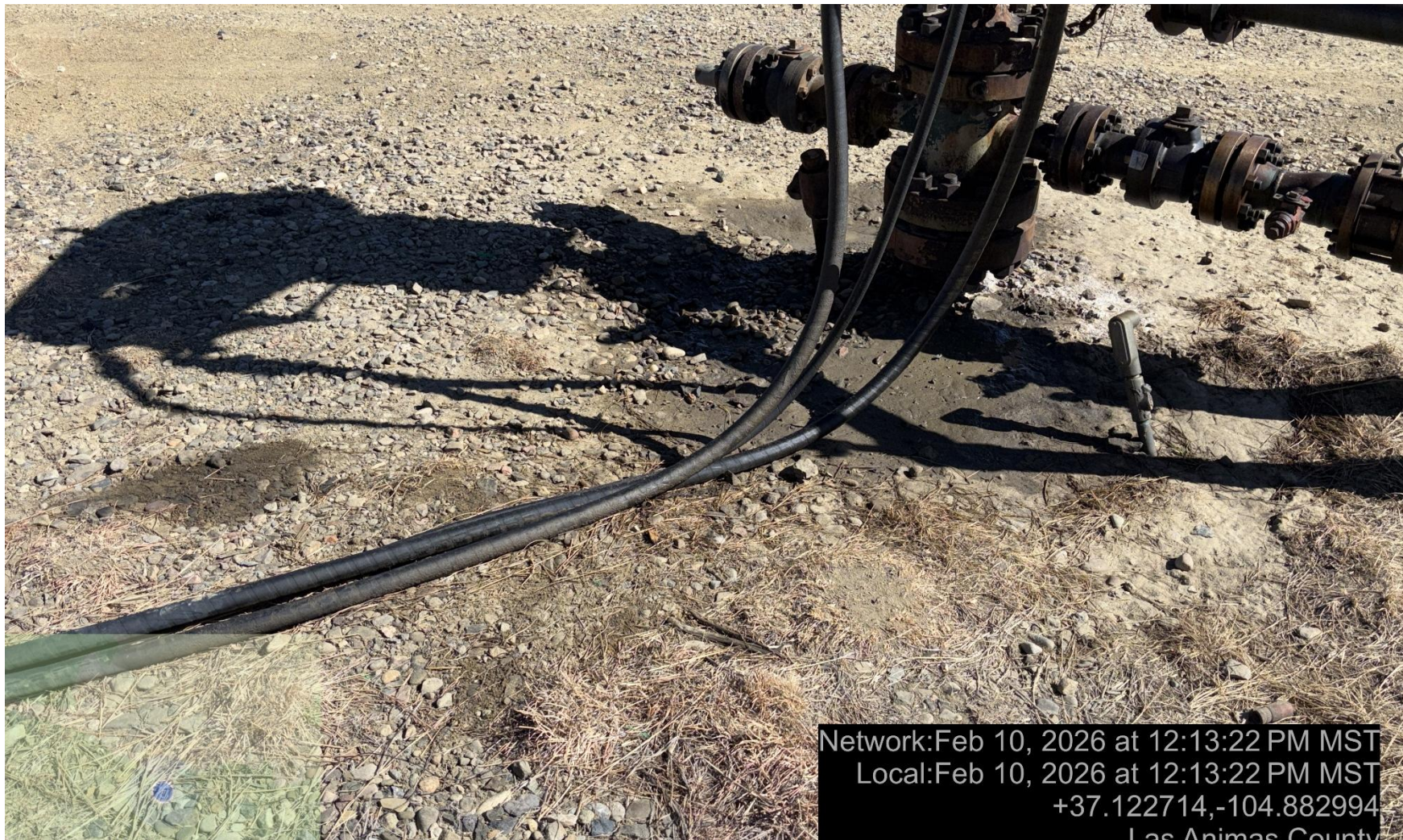
PHOTO 4: area of impacted soil near wellhead appears to be from leaking hydraulic hoses. Conduct maintenance on equipment, cleanup stained material and review self inspection processes. COMPLY WITH RULE 1002,(2).D. ca date 2/23/2026.
