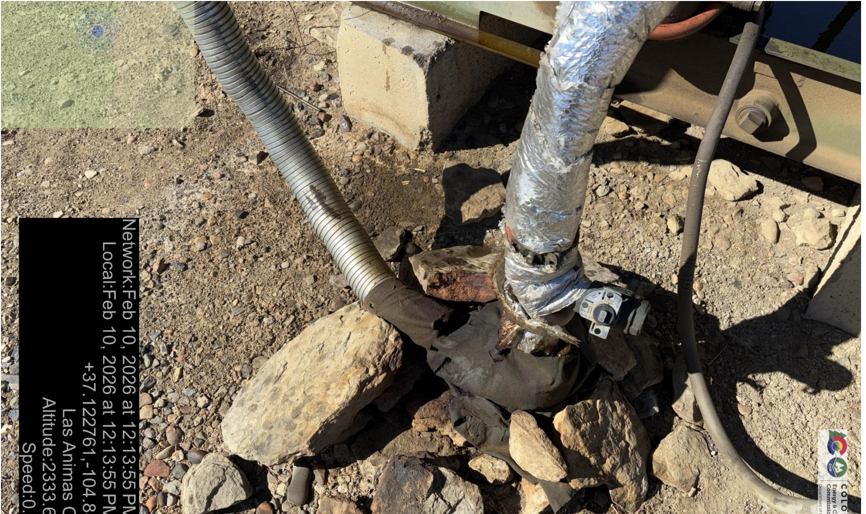
PHOTO 5: area of impacted soil near prime mover skid appears to be used oil leaking out of exhaust. Conduct maintenance on equipment, cleanup stained material and review self inspection processes. COMPLY WITH RULE 1002,(2).D. ca date 2/23/2026.
