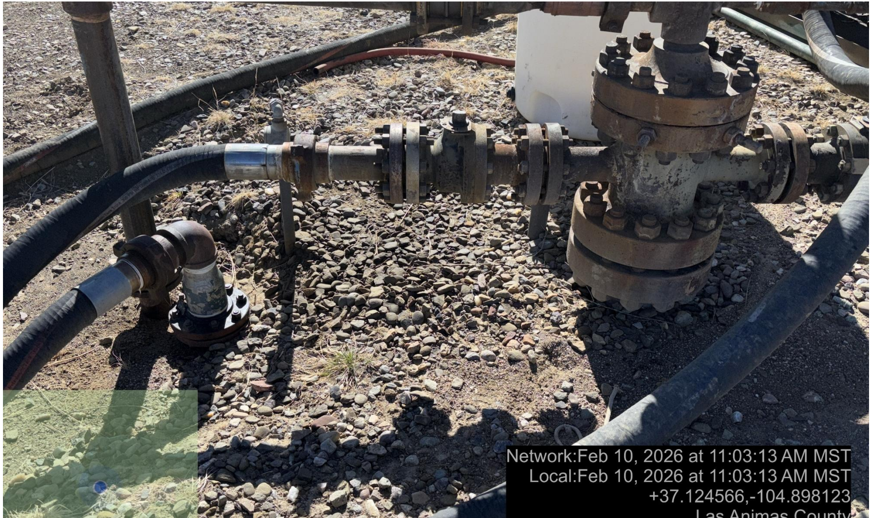
PHOTO 5: Area of impacted soil near wellhead. Conduct maintenance on equipment, cleanup stained material and review self inspection processes. COMPLY WITH RULE 1002,(2).D. ca date 2-27-2026.
