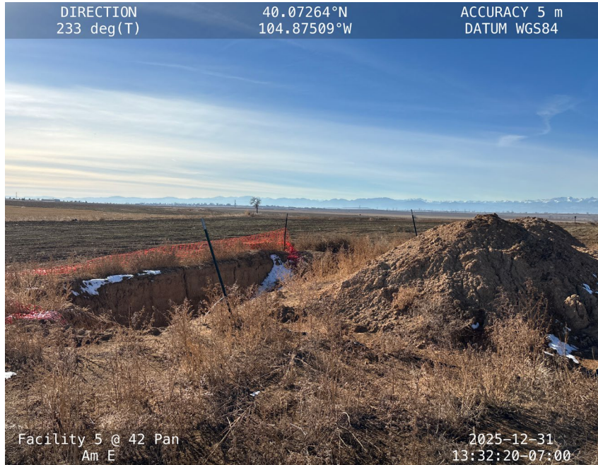
Excavation. Torn fencing, weeds. Stockpile with no stormwater BMPs
