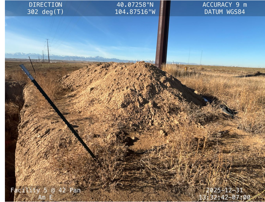
Stockpile with no stormwater BMPs
