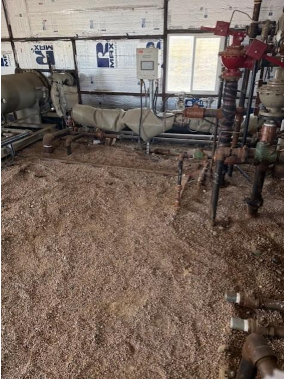
Photo #7 Motu East 28-21-16-1CH Stained Soil Cleaned up
