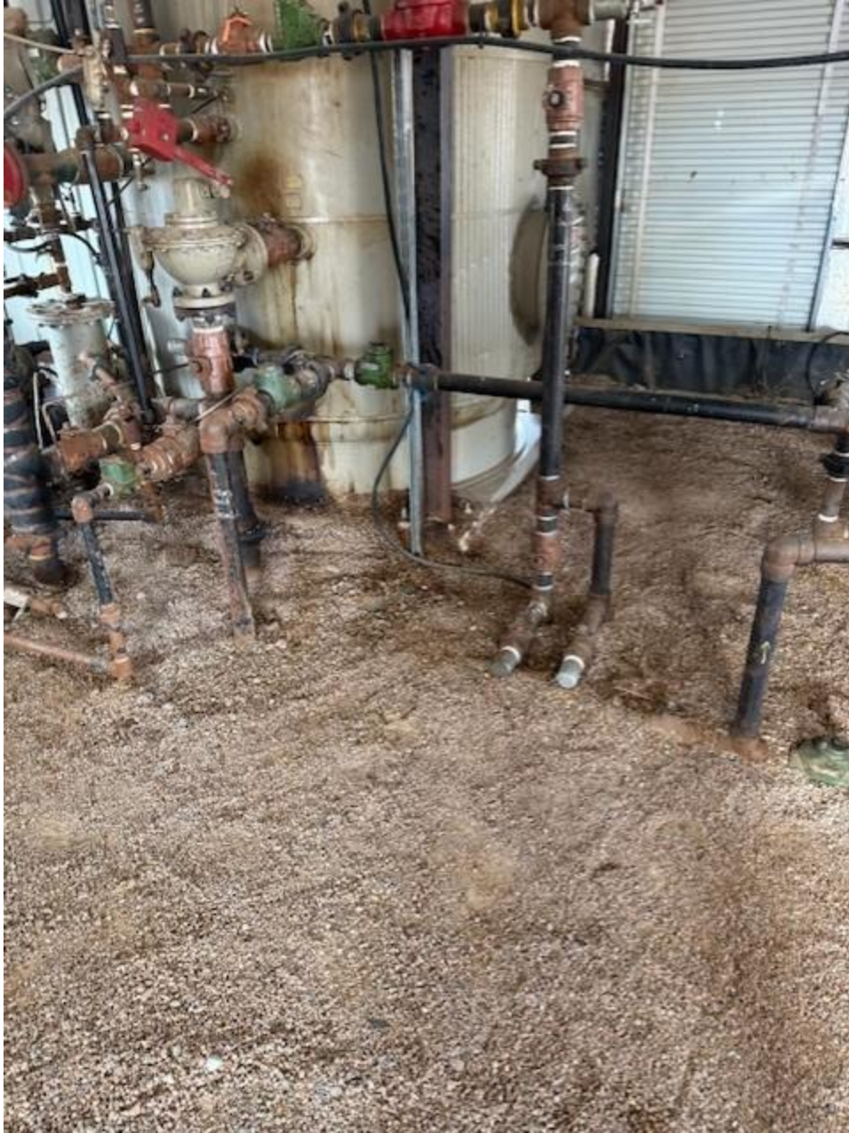
Photo #8 Motu East 28-21-16-1CH Stained soil cleaned up
