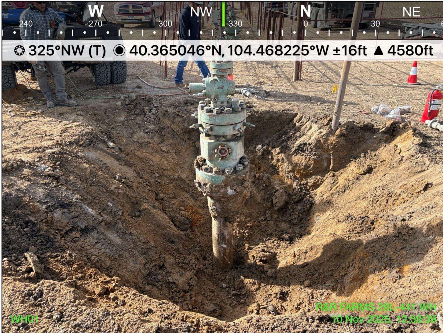
Photo 5: View of excavation extent, facing northwest
