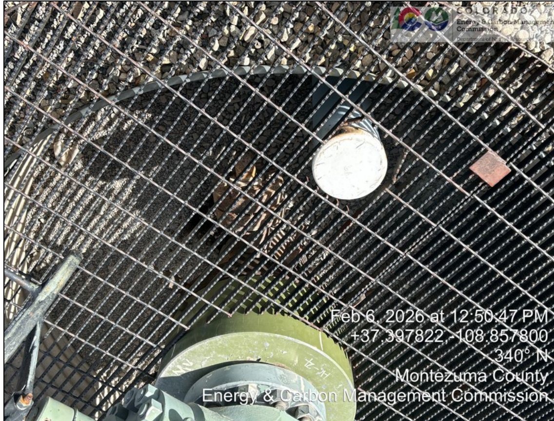
04. Bradenhead access beneath metal grating atop well cellar.
