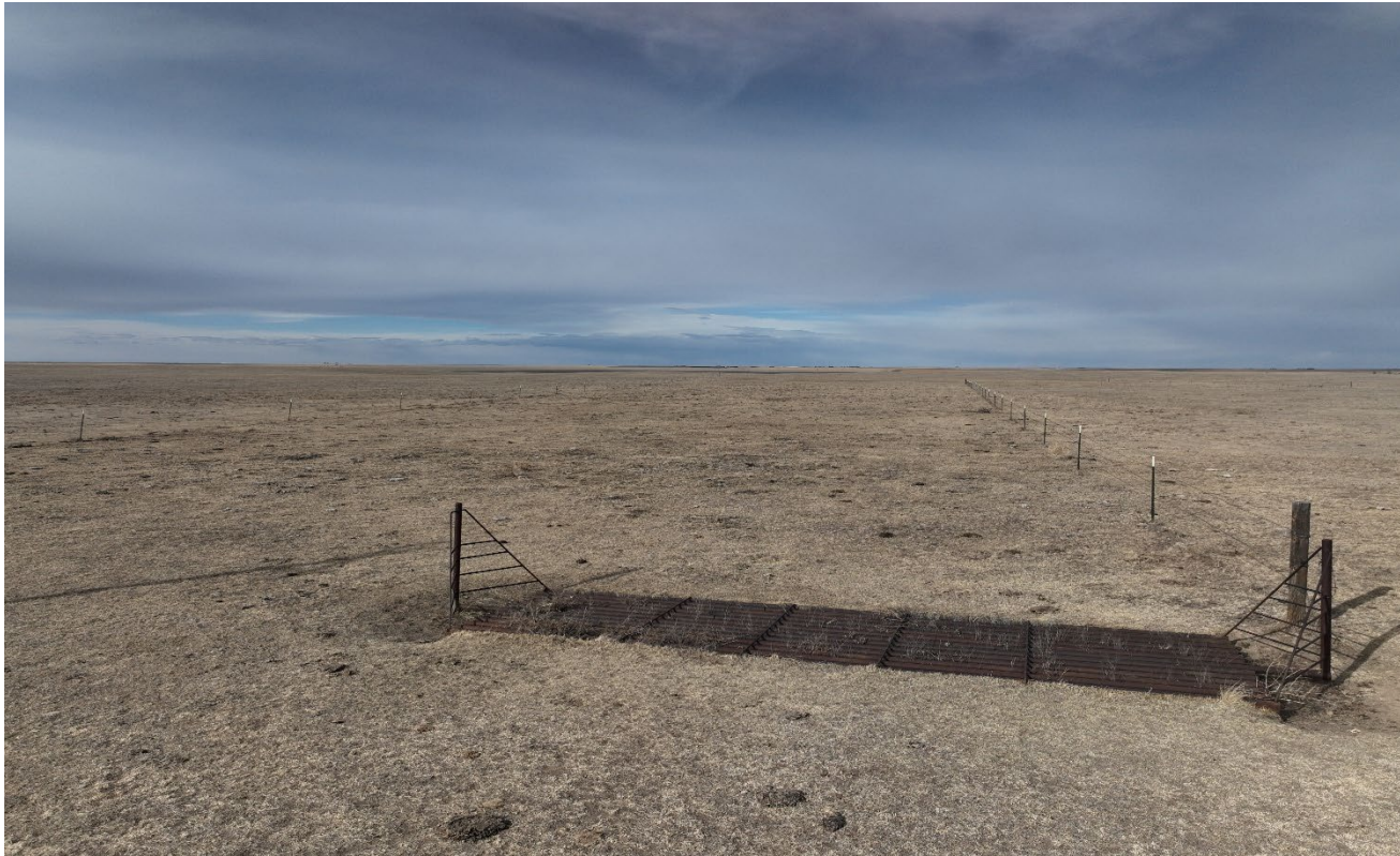
Photo 1. Facing north at the beginning of the former access road. The cattleguard and perimeter fence have not been removed.
