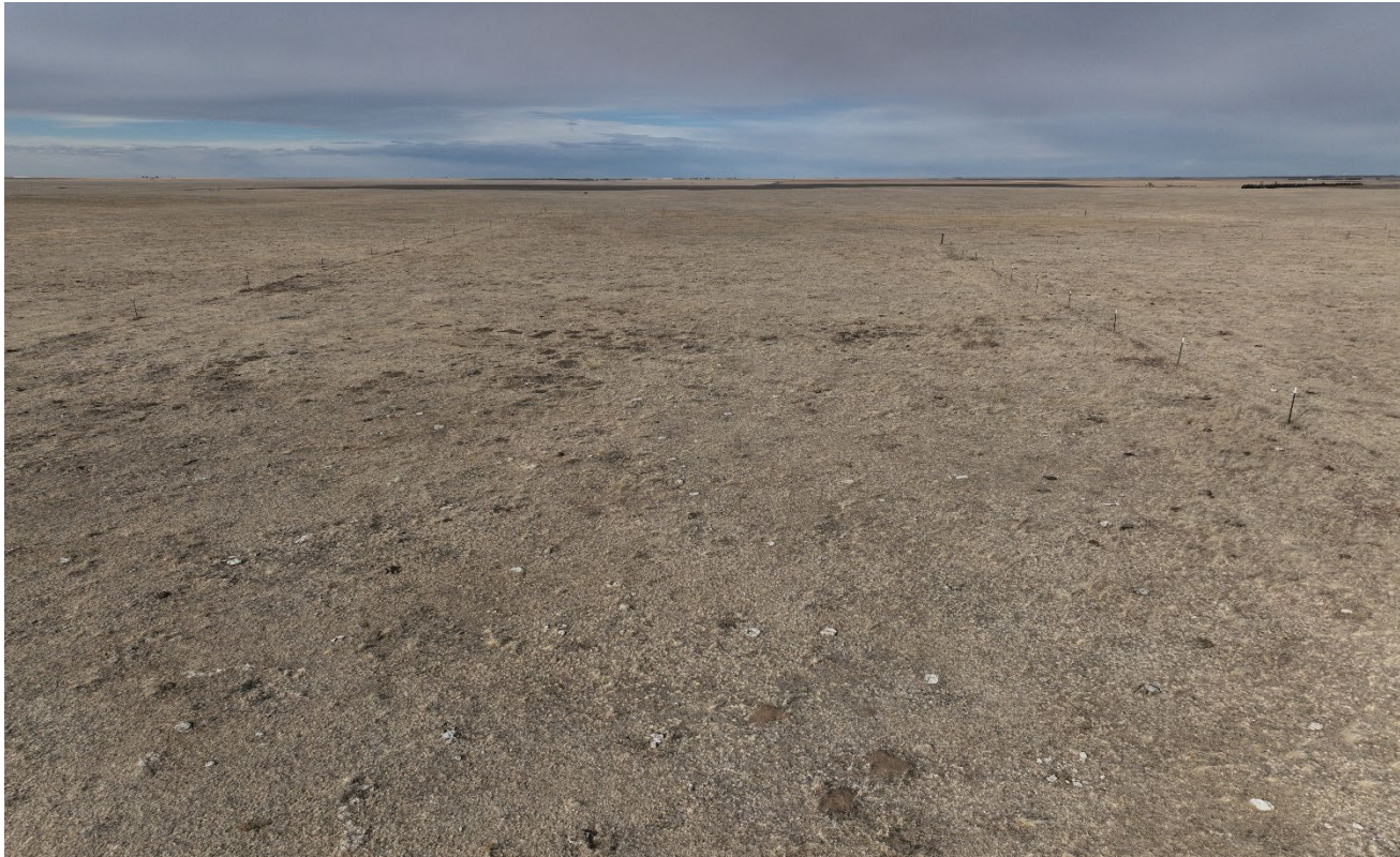
Photo 2. Facing east at the location . The perimeter fence remains around the location and is in disrepair.
