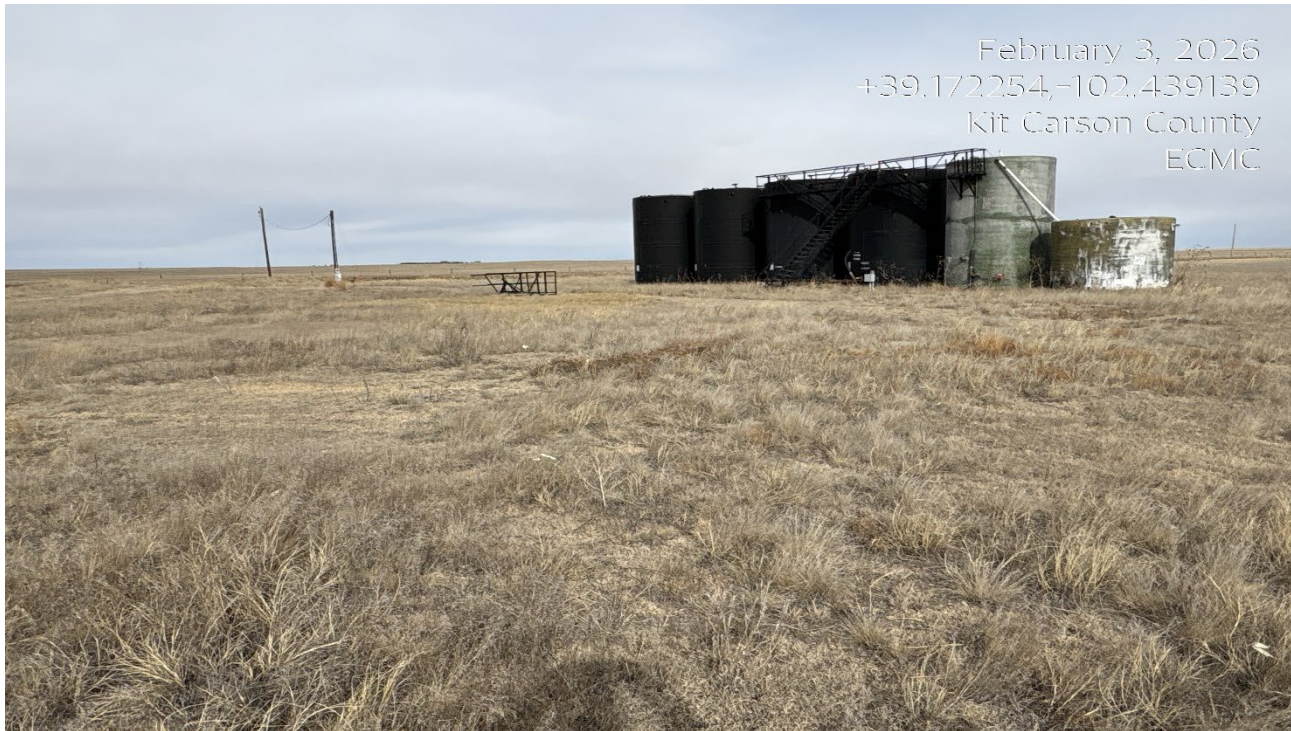
Photo 2. Tank battery was not removed. All equipment should have been removed within 3 months of abandonment..
