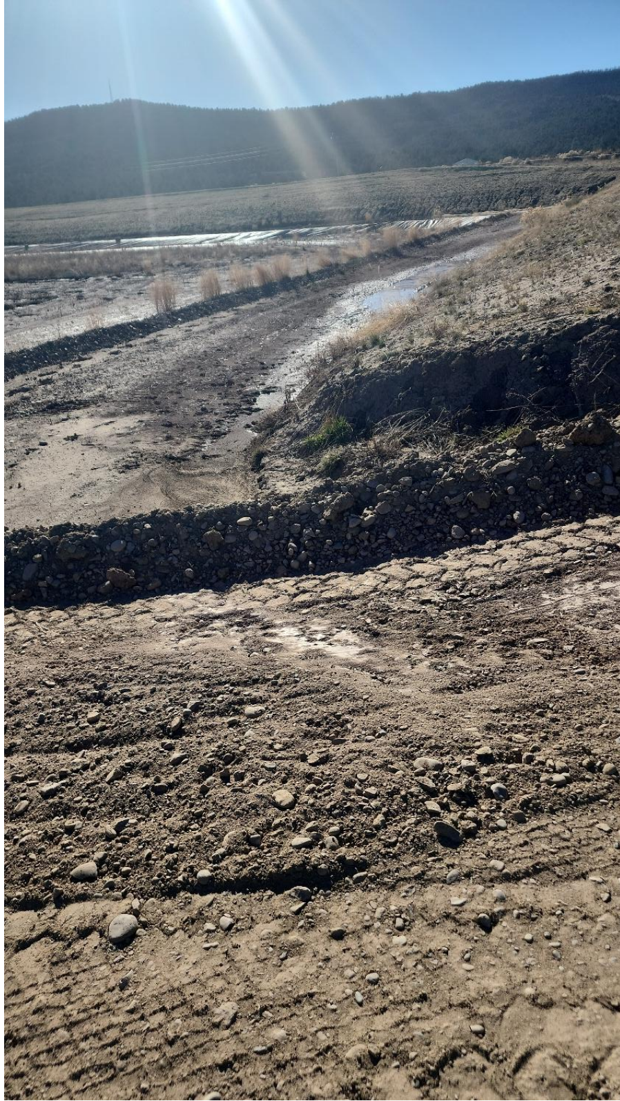
Photo 12: November 11, 2026. Drainage berms re-established. Post Repair.
