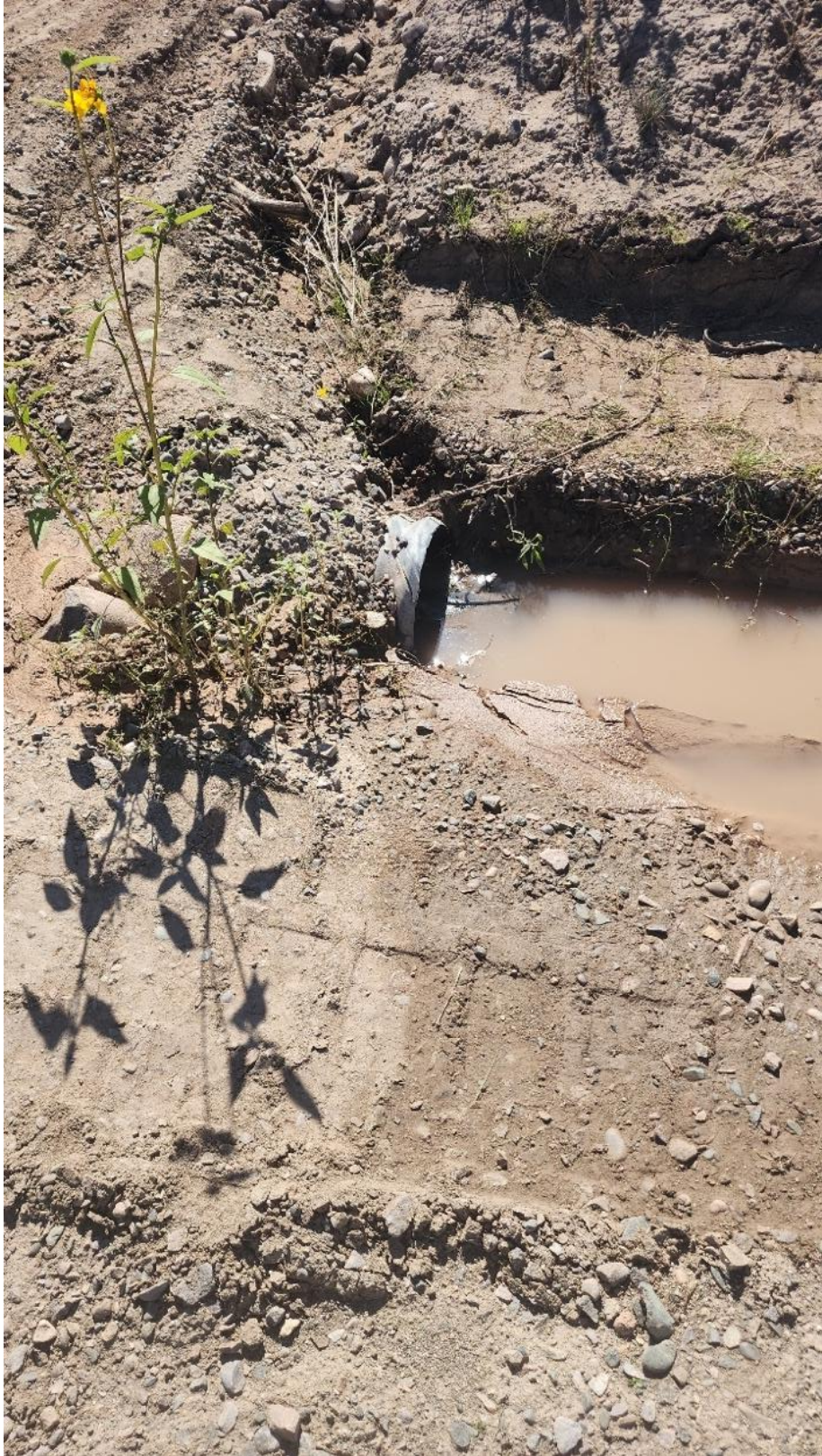
Photo 8: November 11, 2025. Repaired culver. Post Repair.
