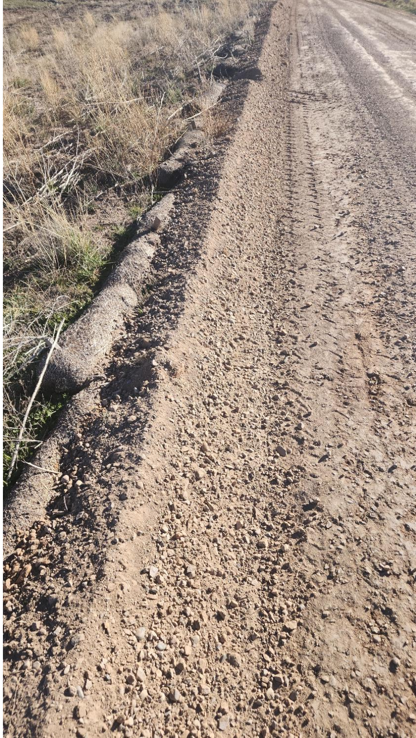
Photo 14: November 11, 2025. Straw Wattles realigned along access road. Post Repair.
