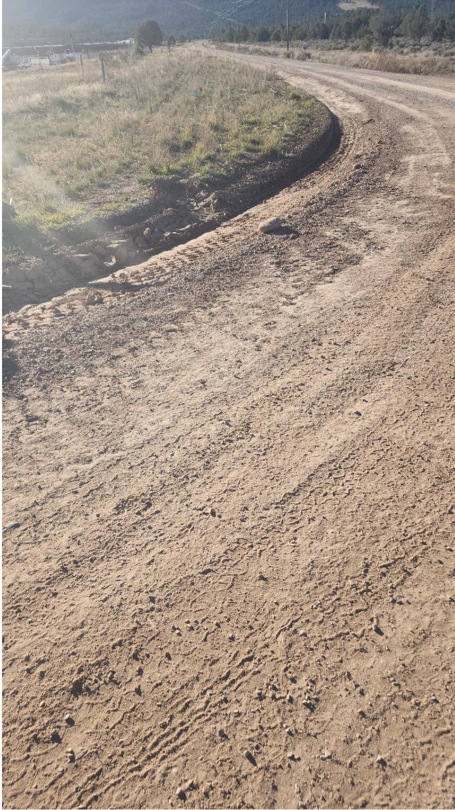
Photo 10: November 11, 2025. Well pad access road, graded and drainage re-established. Post Repair.
