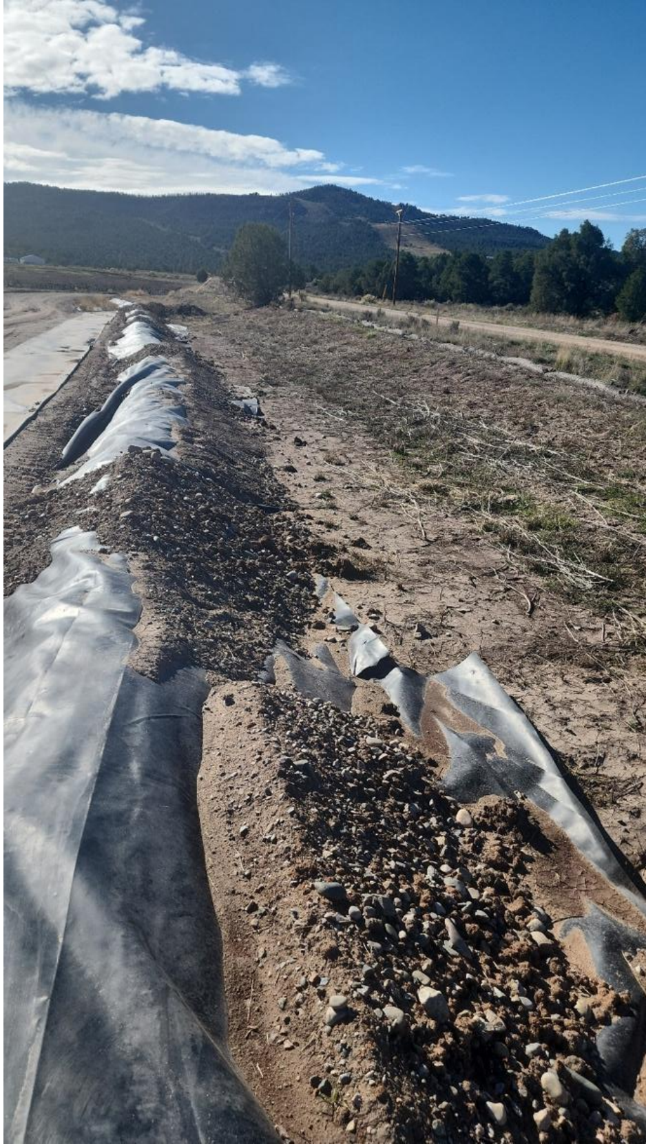
Photo 4: September 26, 2025. Bermed liner, sandbags removed, west side of TUA. Post Repair.
