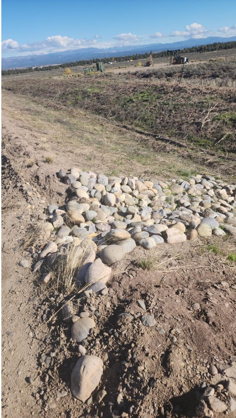
Photo 2: October 24, 2025. Access road east of TUA. Post Repair.
