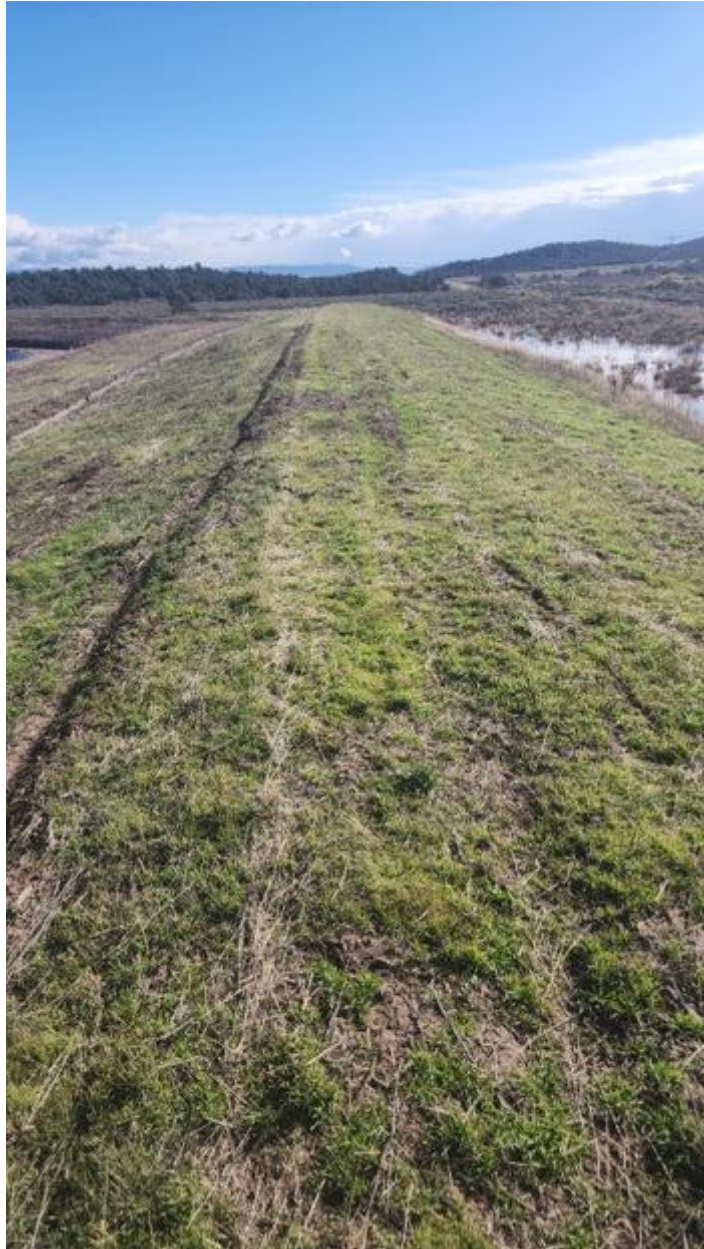
Photo 5: October 24, 2025. Looking east along Topsoil Stockpile #1 at area post treatment.
