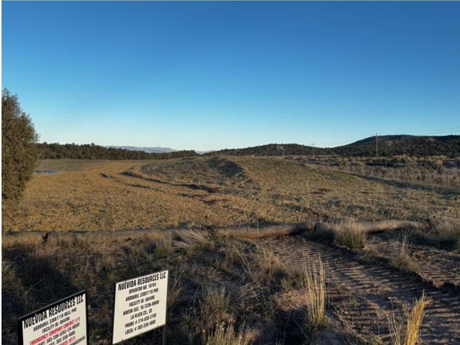
Photo 6: November 15, 2025. Looking east at Topsoil Stockpile #1. Post hydro-mulch reseeding.
