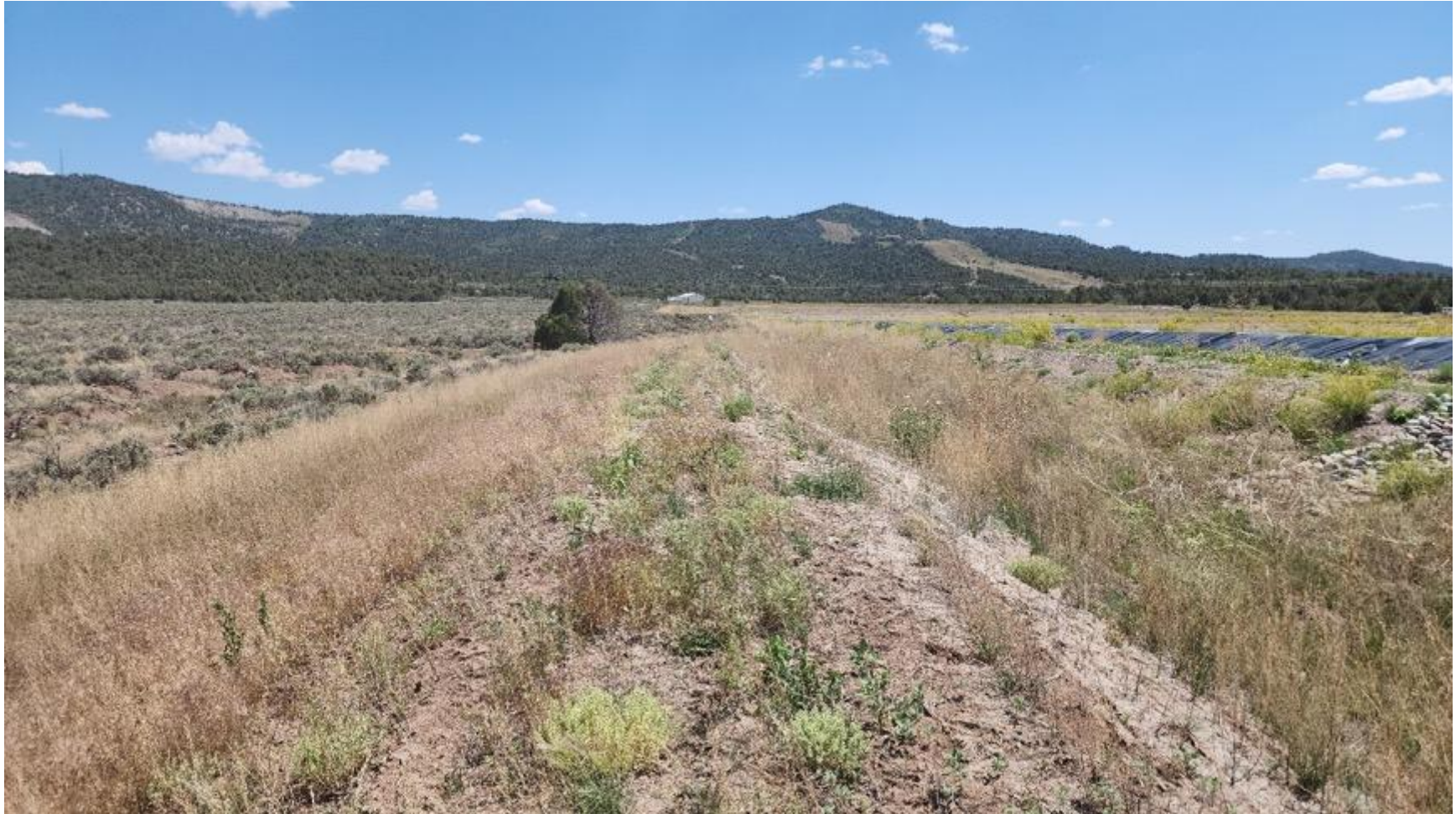
Photo 7: June 12, 2025. Looking south-southwest along Topsoil Stockpile #2. Post herbicide application, pre mechanical treatment.
