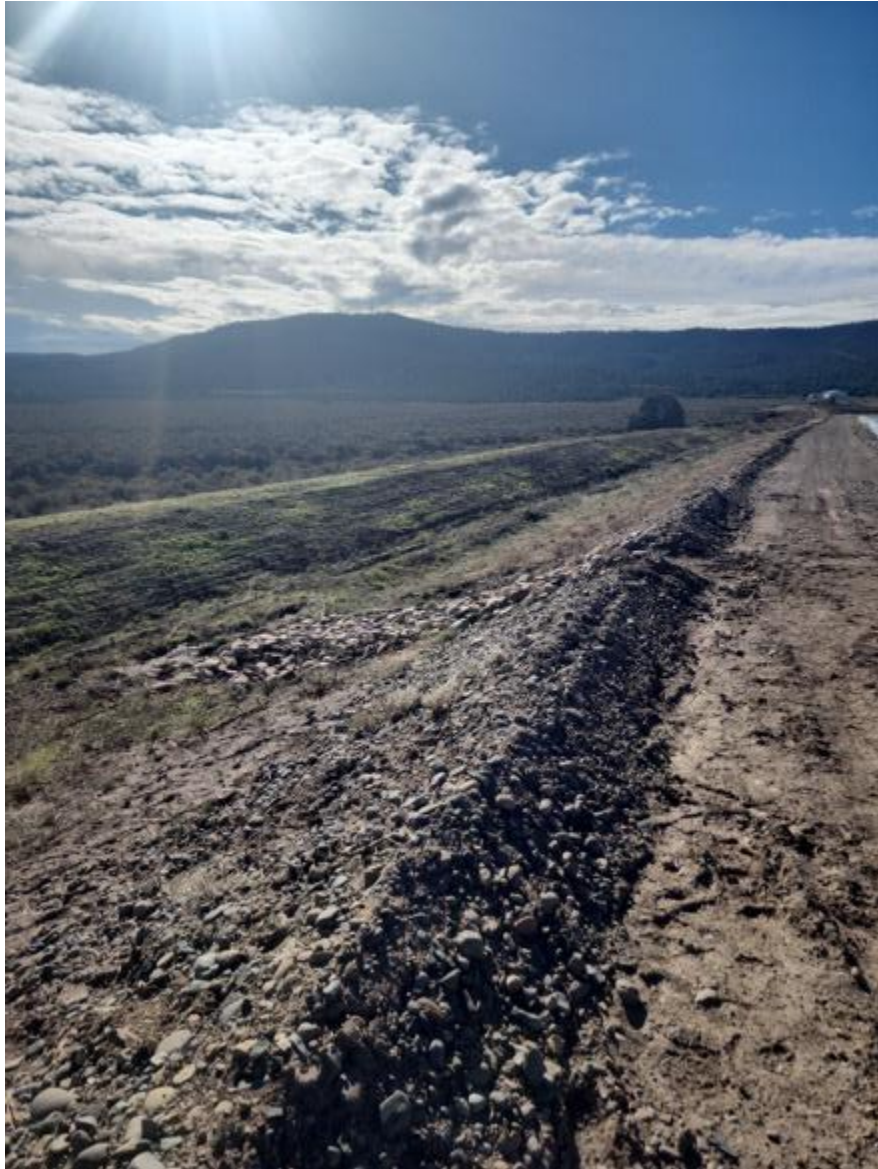
Photo 8: October 24, 2025. Looking south-southwest at Topsoil Stockpile #2. Post treatment.
