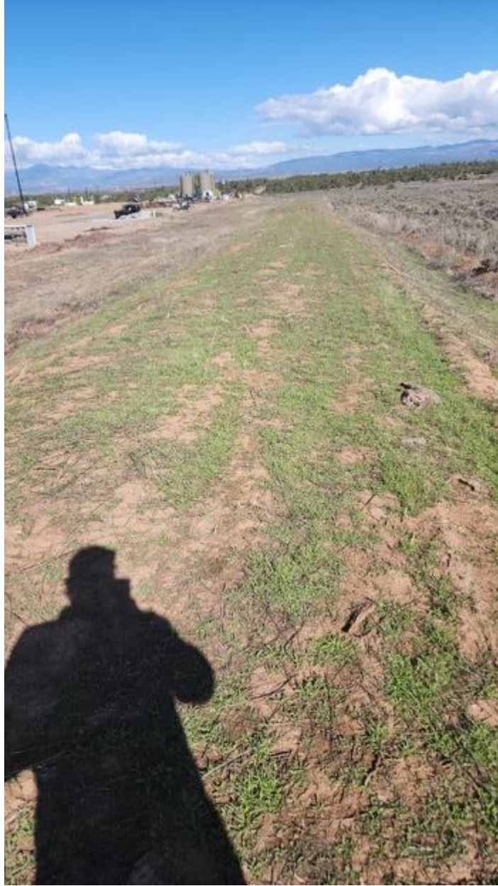
Photo 10: October 24, 2025. Looking north along Topsoil Stockpile #3. Post treatment.
