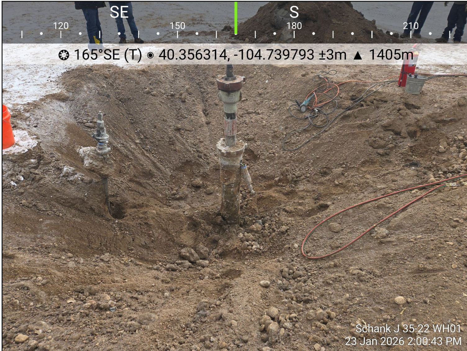
Photo 3: View of excavation extent, facing south-southeast
