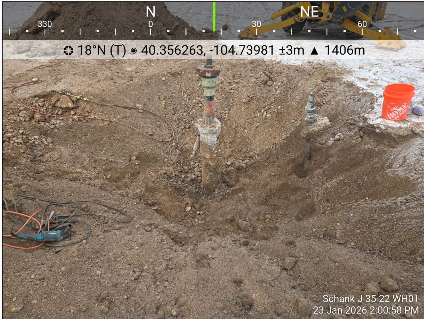
Photo 1: View of wellhead excavation extent, facing north-northeast
