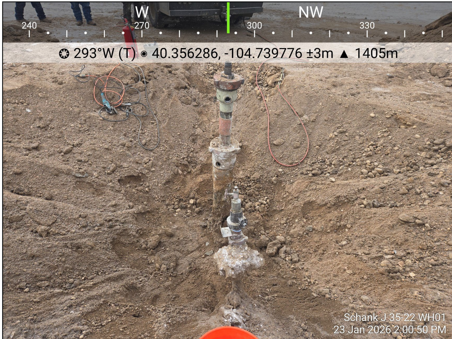
Photo 2: View of wellhead excavation extent, facing west-northwest
