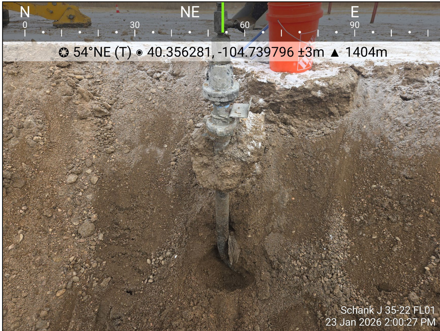
Photo 5: View of FL01-R-W sample location inside excavation extent, facing northeast
