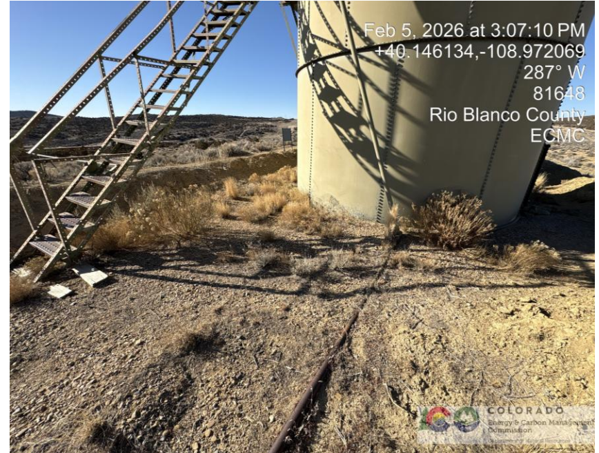
Photo # 1795 Weeds/undesirable plant species presents a potential fire hazard
