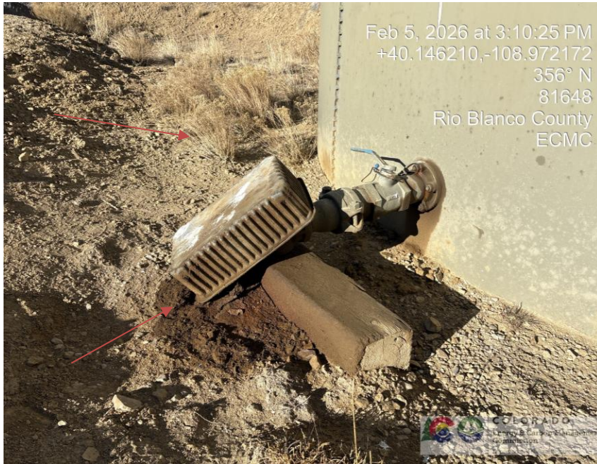
Photo # 1800 Staining/Weeds/undesirable plant species presents a potential fire hazard
