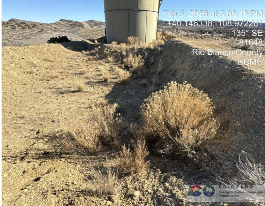
Photo # 1796 Weeds/undesirable plant species presents a potential fire hazard
