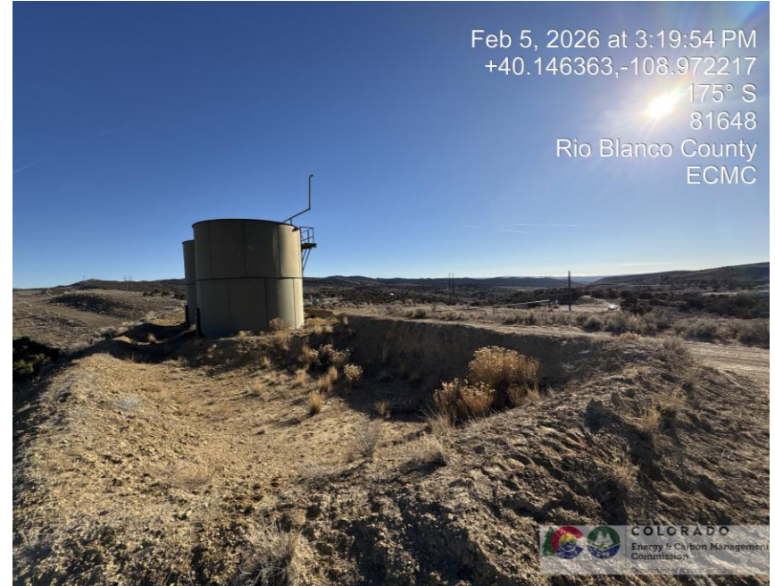
Photo # 1819 NW corner of location
