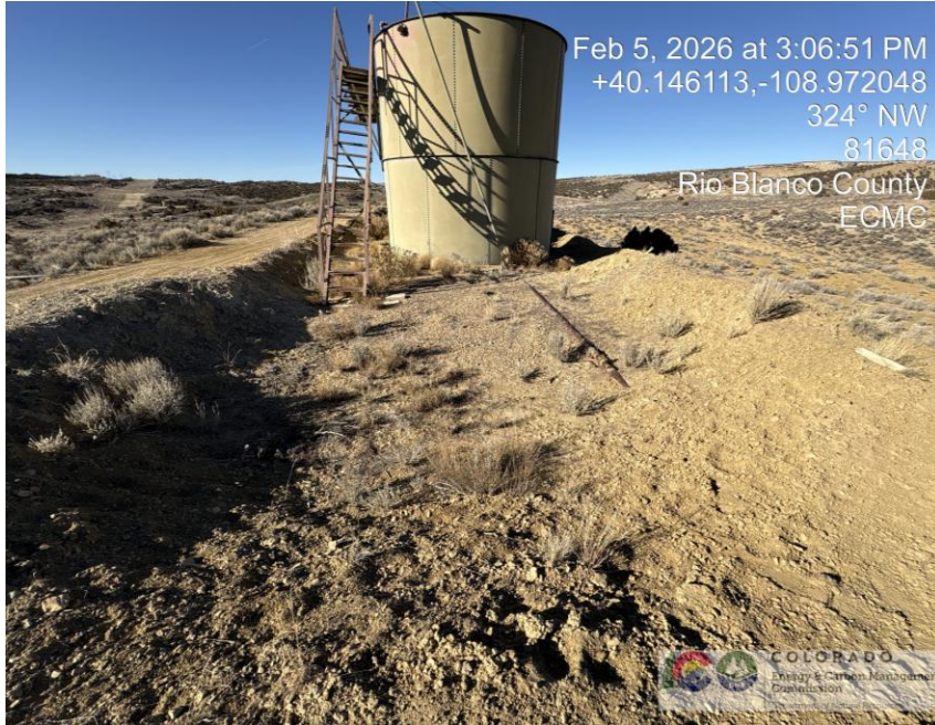
Photo # 1794 Weeds/undesirable plant species presents a potential fire hazard
