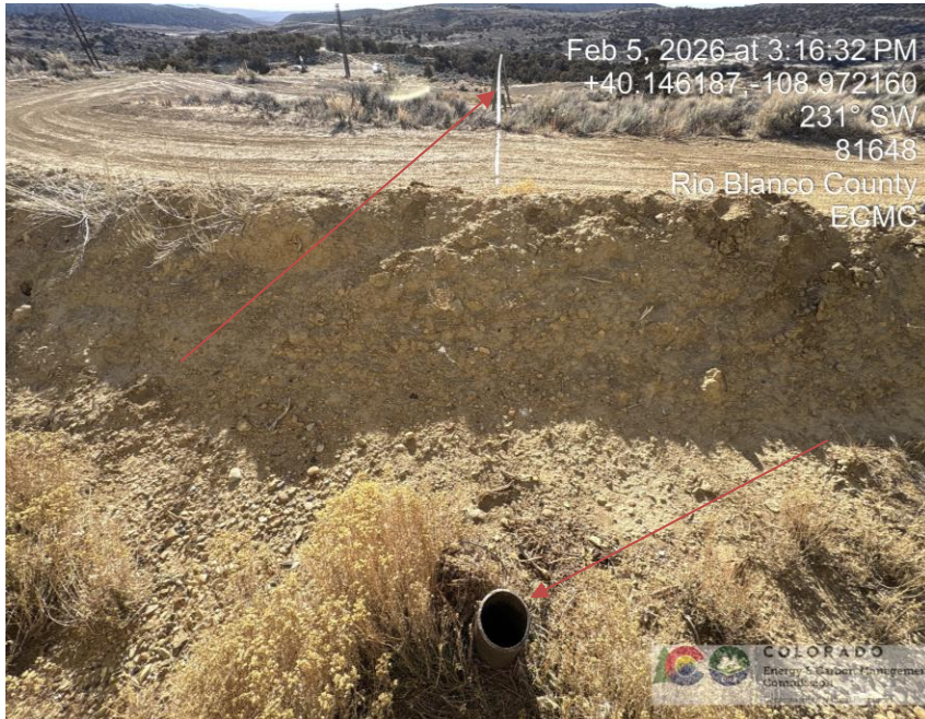
Photo # 1815 Unused unload line near tank battery not necessary for use on location
