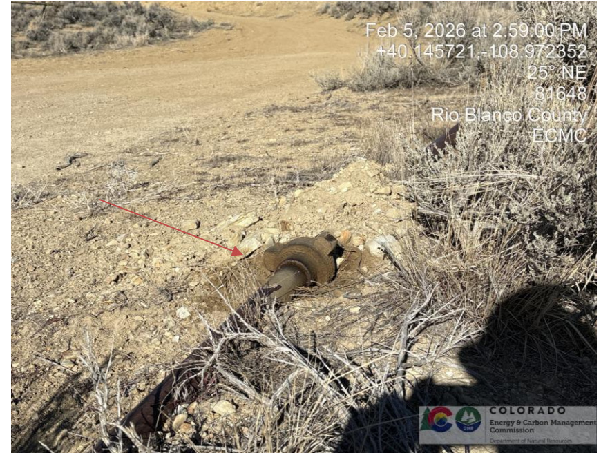
Photo # 1785 Staining/Weeds/undesirable plant species presents a potential fire hazard
