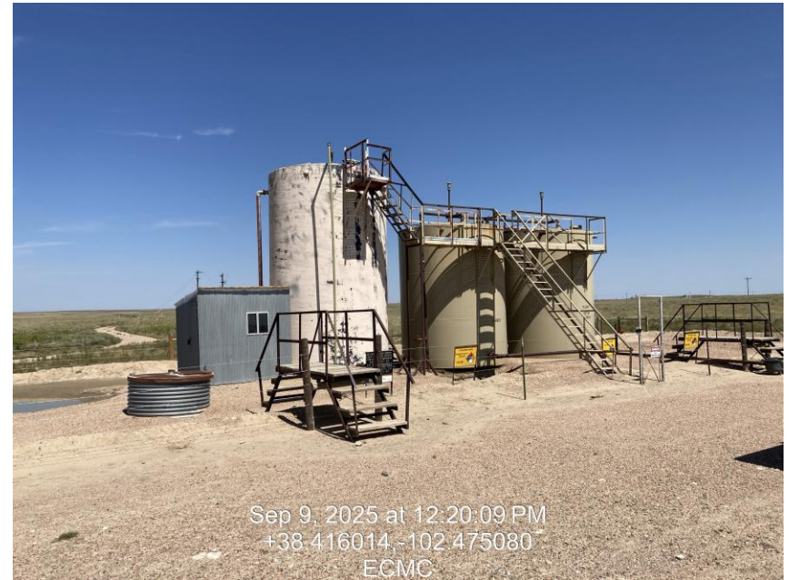
Photo 2 – Tank Battery
