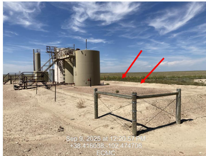
Photo 6 – Unused Tanks removed
