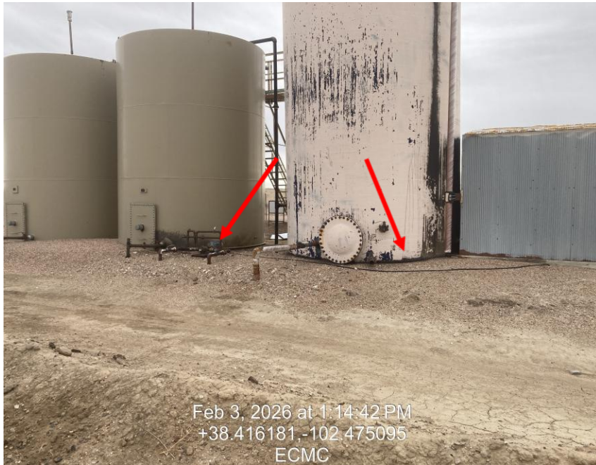
Photo 7 – Impacts to soil at tank base
