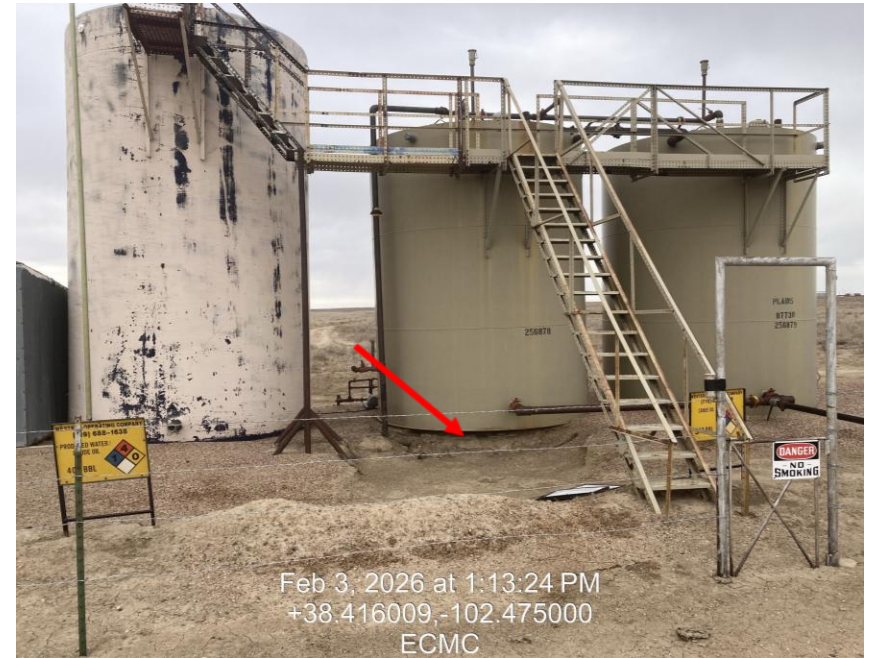
Photo 2 – Tank Battery open excavation
