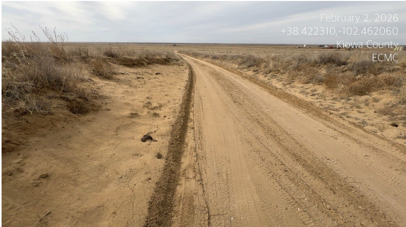
Photo 4. Facing back to the west. The sandy soils are susceptible to further erosion. This area needs to be repaired and stabilized.
