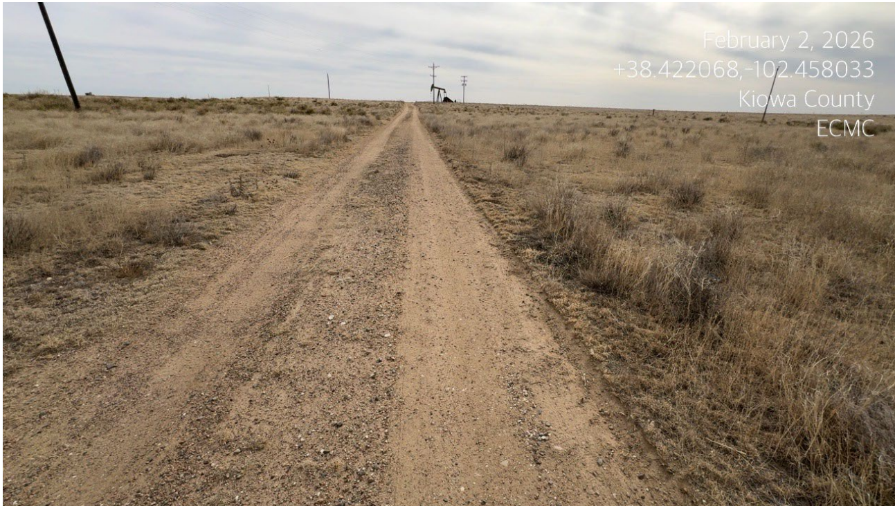
Photo 5. Facing south along the access road.
