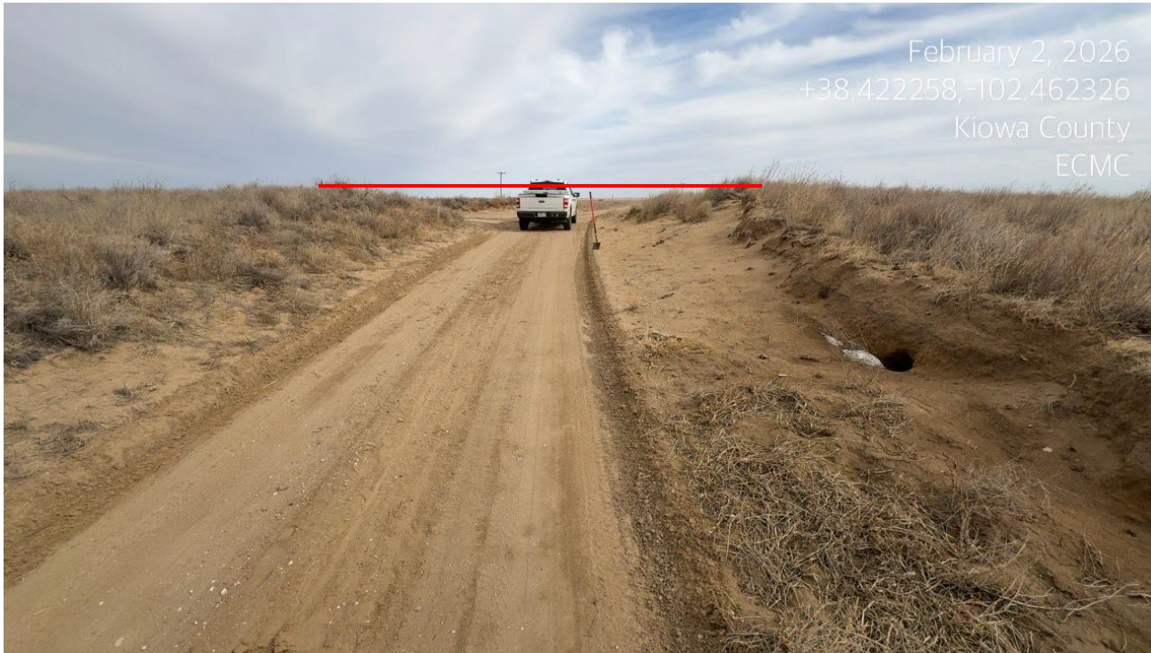
Photo 2. Facing east along the main access road. Red line is the approximate original grade and the shovel is 4.5 feet for scale. There is concern for winter snow to blow onto the road impeding vehicle passage.
