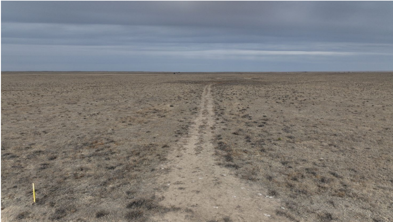
Photo 2. Drone aerial photo facing north. The road has not revegetated and must be reclaimed.
