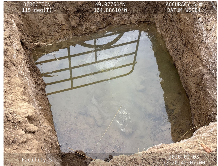
Presumed release point location excavation. Oily sheen observed on water within excavation.
