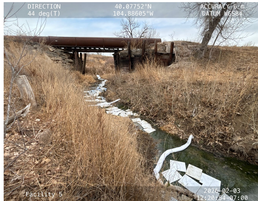
Absorbent mats downstream
