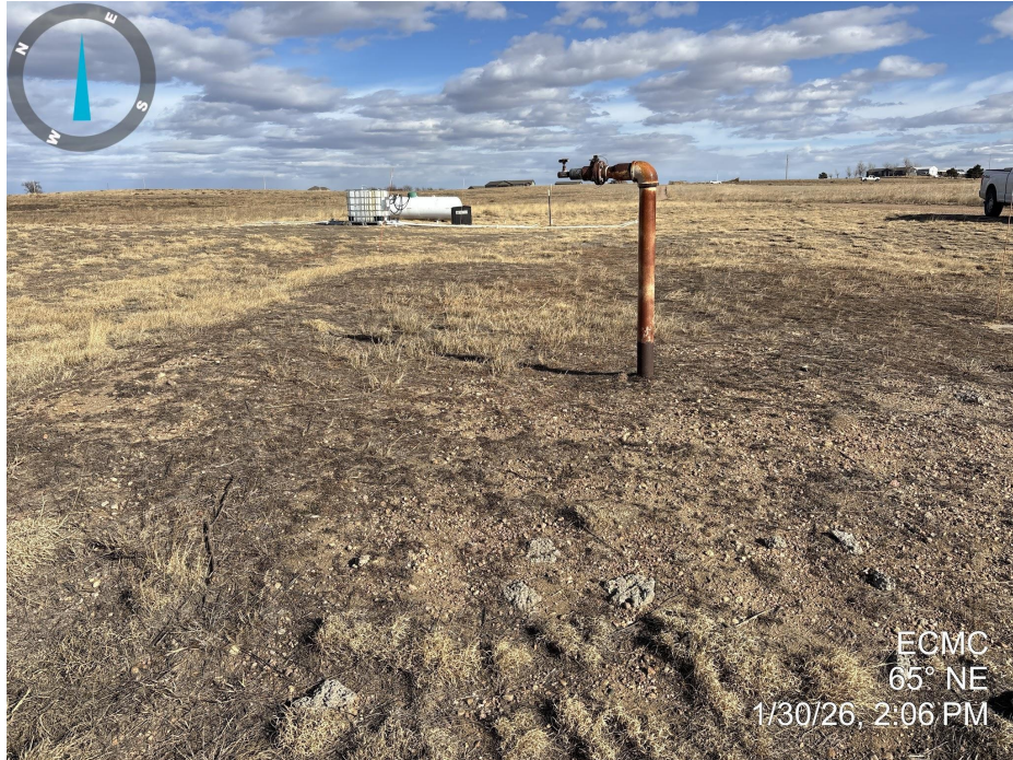
Photo 3. Photo taken of the tank battery location, facing northeast. Photo illustrates equipment remains on the location.
