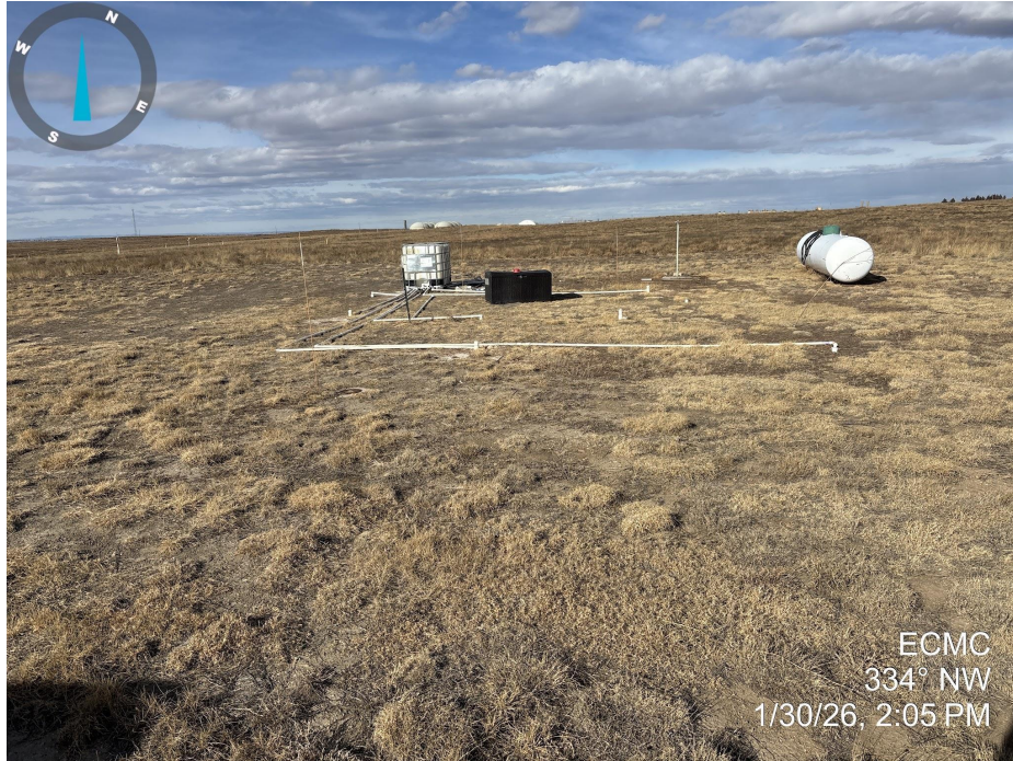
Photo 1. Photo taken of the tank battery location, facing northwest. Photo illustrates that final reclamation activities have not taken place and there is active remediation at the location.
