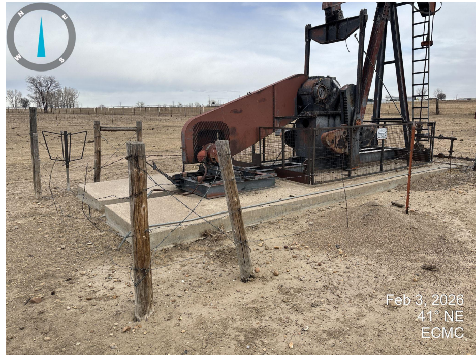
Photo 6. Looking north towards the pumpjack.
