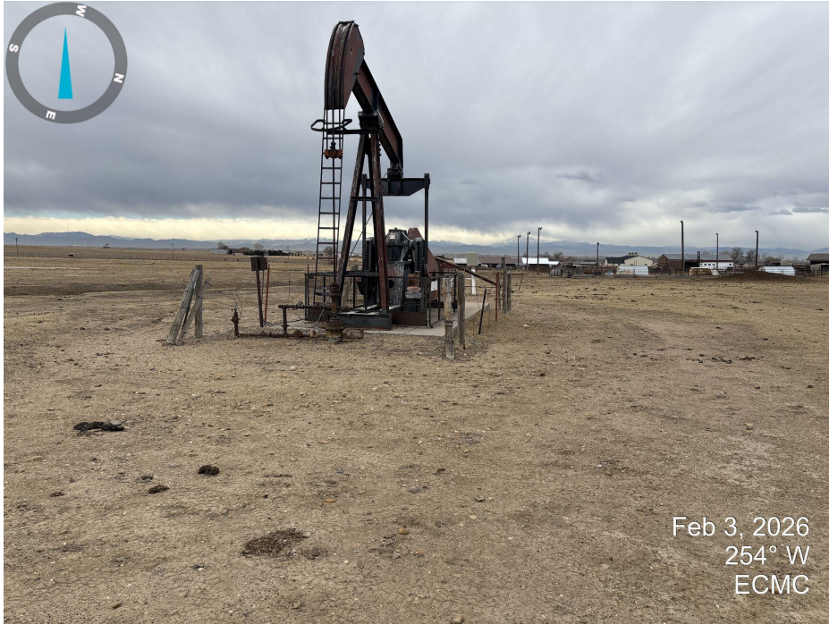
Photo 1. Looking west across the location. The well is in a heavily grazed cattle pen. The location size is appropriate. Weeds are controlled at the time of inspection.
