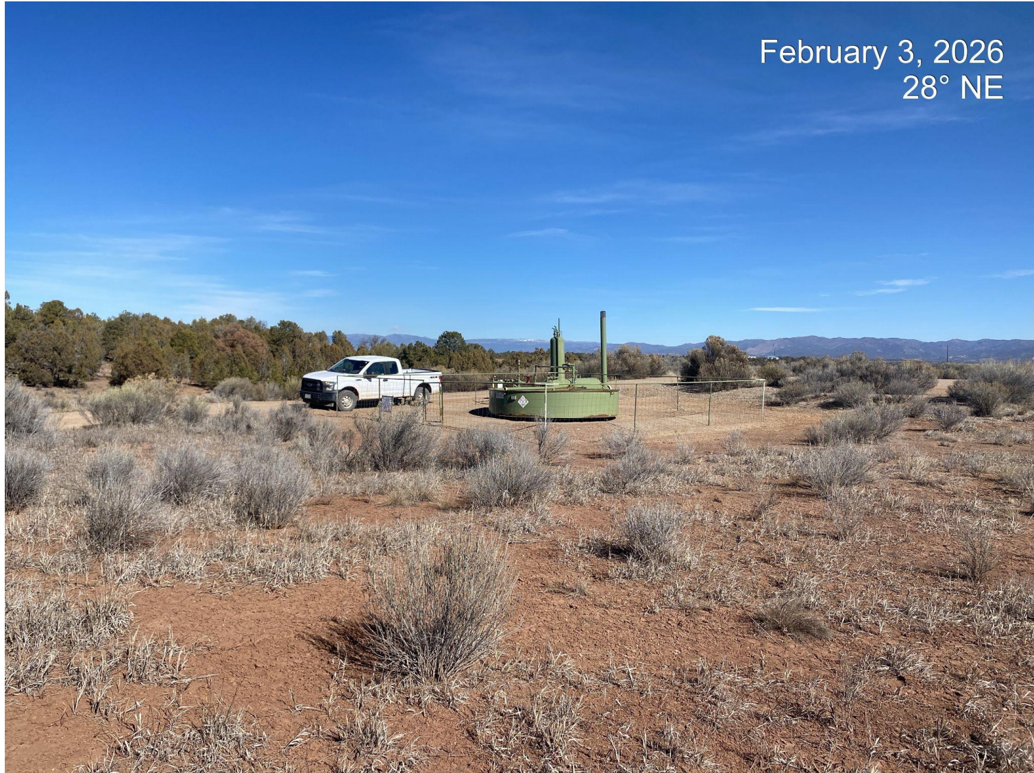
Photo 1. View of the active pad taken from the southern edge facing center.
