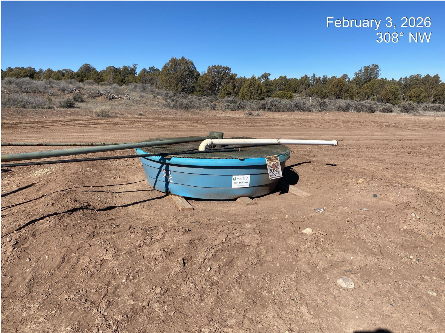
Photo 3. Secondary containment walls have sunken in and is no longer sufficient.
