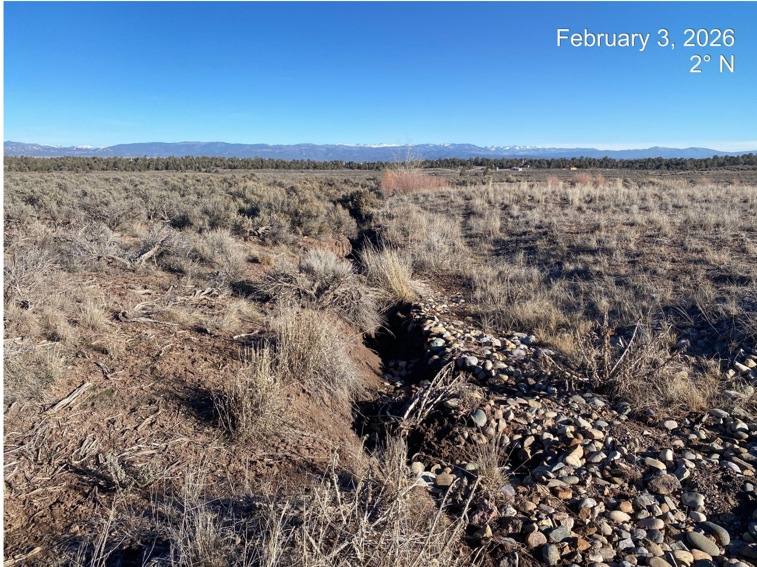
Photo 2. View of gully erosion forming in the NW corner of the disturbance.
