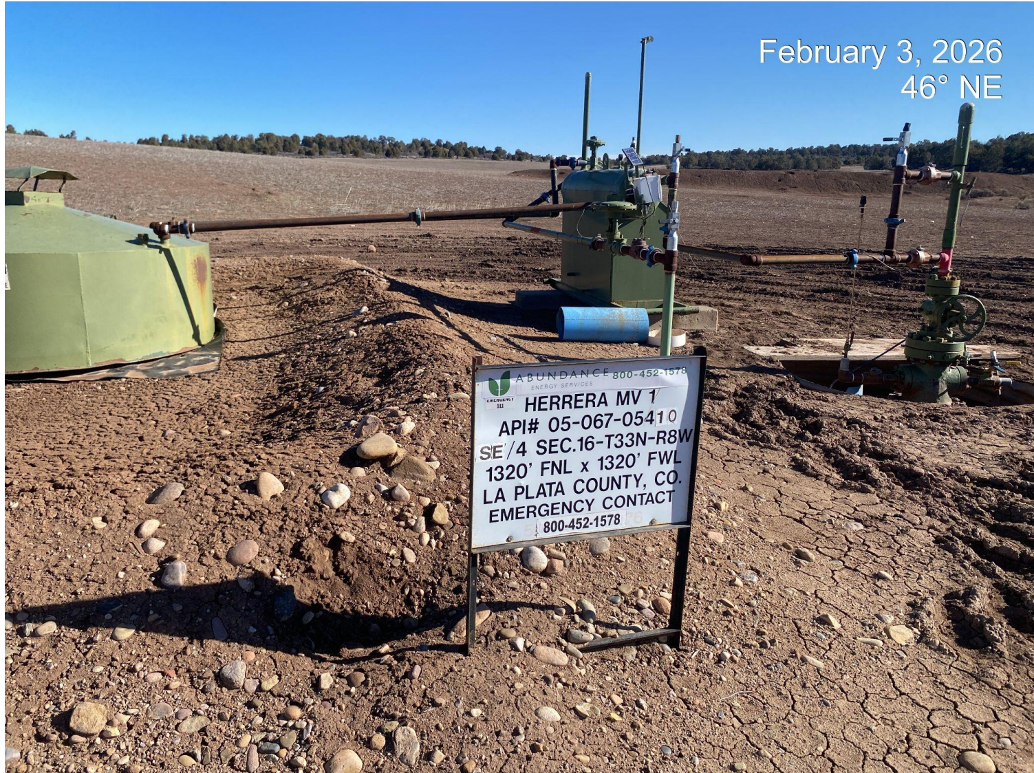
Photo 3. View of wellhead and location sign.
