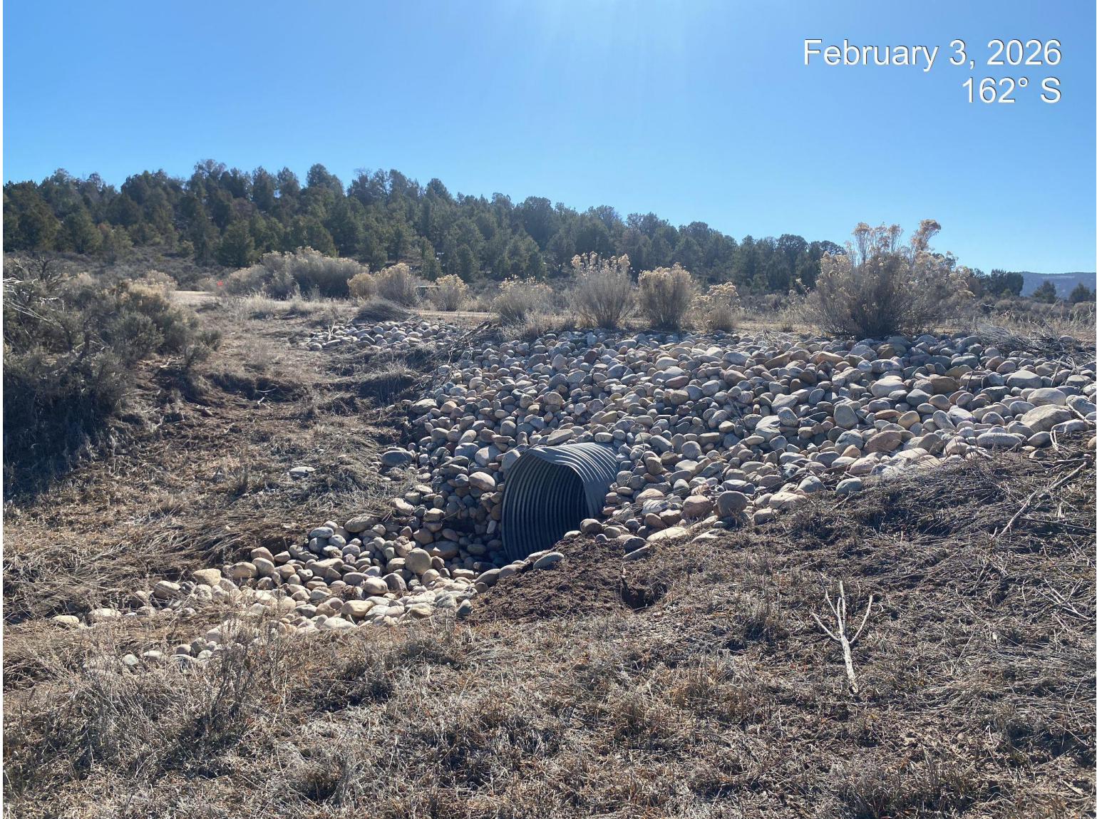
Photo 4. No stormwater issues observed at the culvert along location access point.
