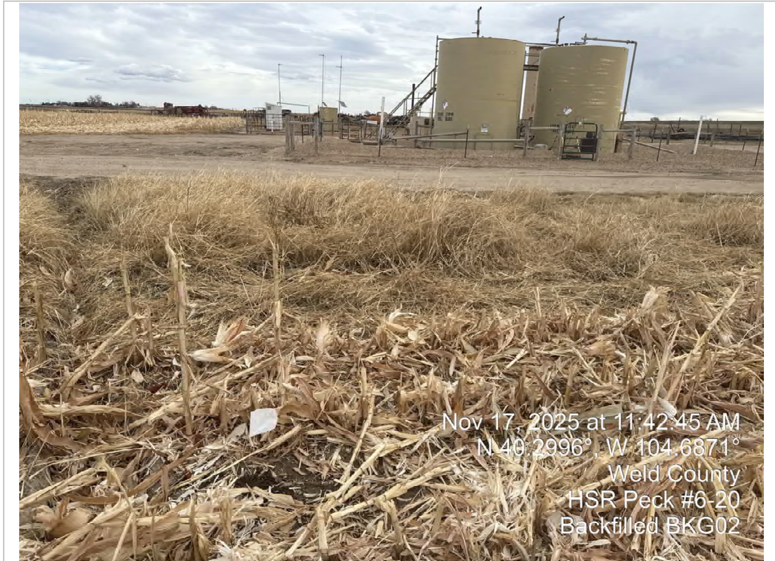
BKG02: View East
