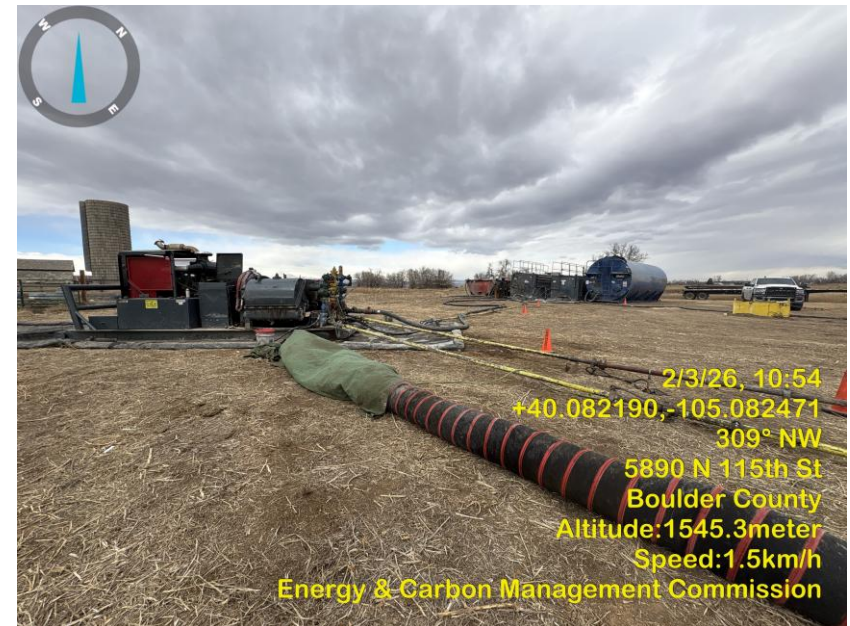
Photo 12 Rig pump, circulation tanks, freshwater tank.
