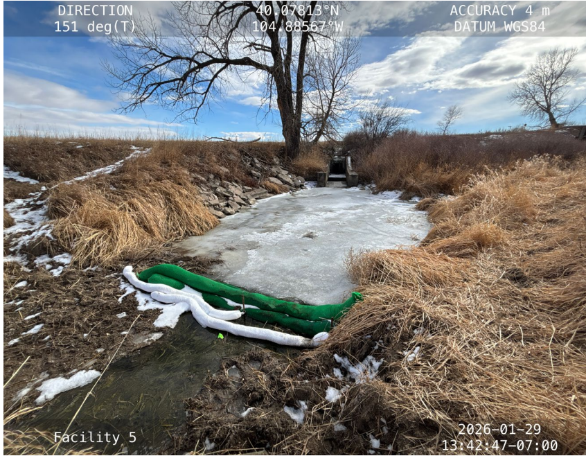
Inadequate booms
