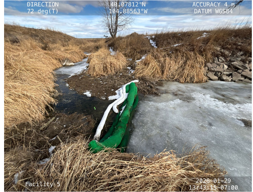
Inadequate booms
