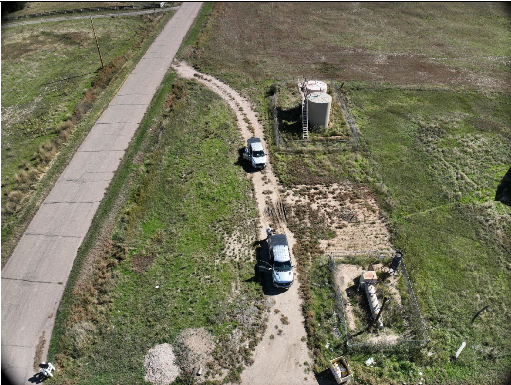
In View – Tank Battery, Separator, Flowlines
