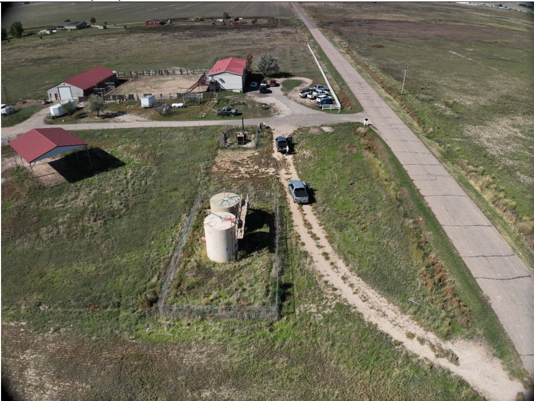
In View – Tank Battery, Separator, Flowlines
