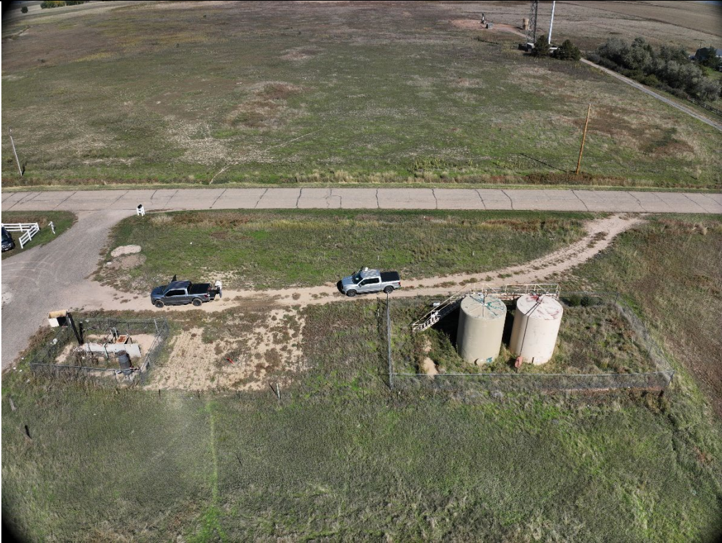
In View – Tank Battery, Separator, Flowlines
