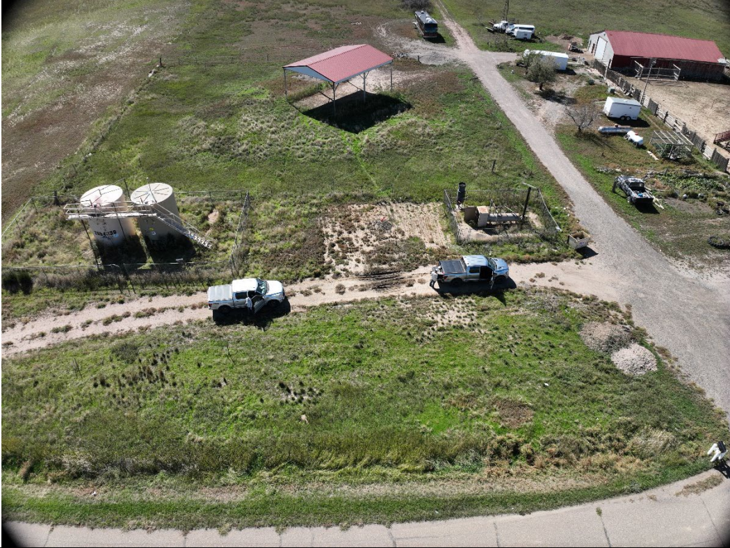
In View – Tank Battery, Separator, Flowlines
