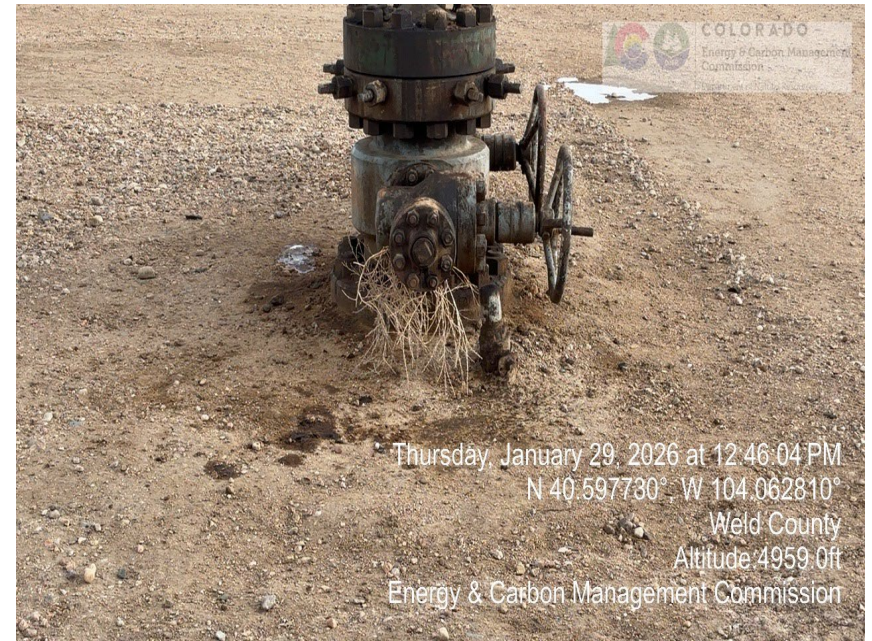
Photo 8 – 2-3H Wellhead – Stained Soil
