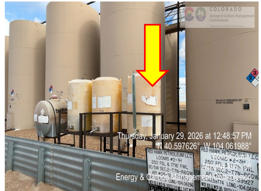
Photo 18 – Chemical Label has faded no longer visible
