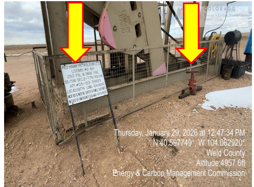
Photo 14 – 2-6H Well Sign - Previous Operator's Info still visible and unused Wellhead Parts
