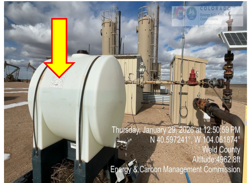
Photo 26 – Label has faded no longer visible
