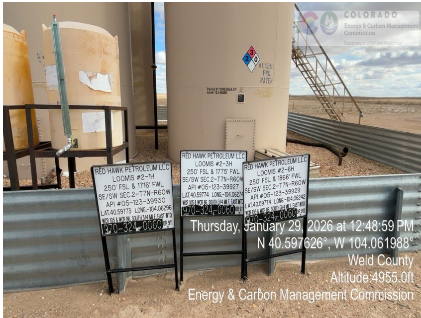
Photo 19 – Tank Battery Signs – Previous Operator's Info still visible
