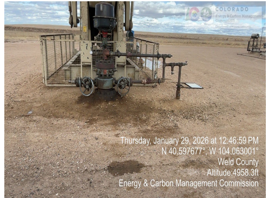
Photo 12 – 2-6H Wellhead – Stained Soil
