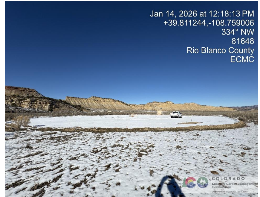
Photo # 1043 SE corner of location
