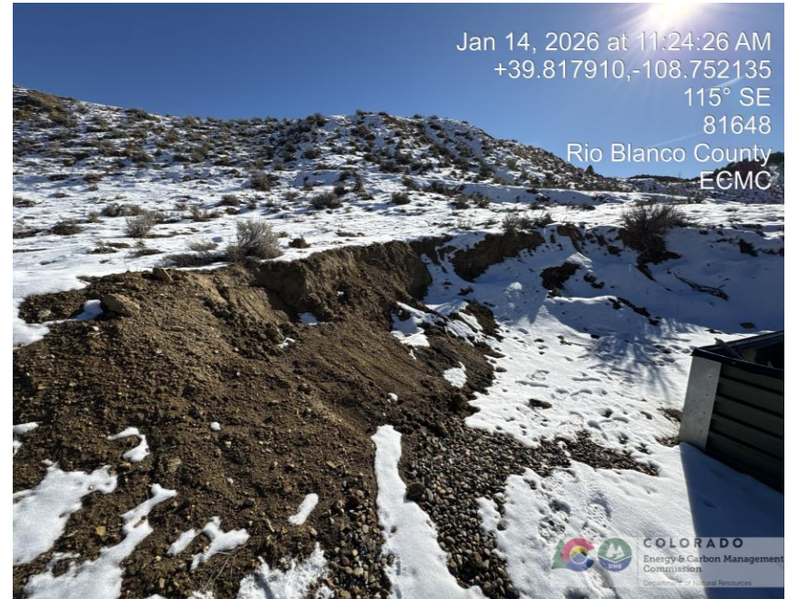
Photo # 1009 Erosion & transport of sediment on cut slope, sediment is migrating onto location near tank battery, the cut slope has experienced progressive erosion and is now actively sloughing, resulting in slope instability.
