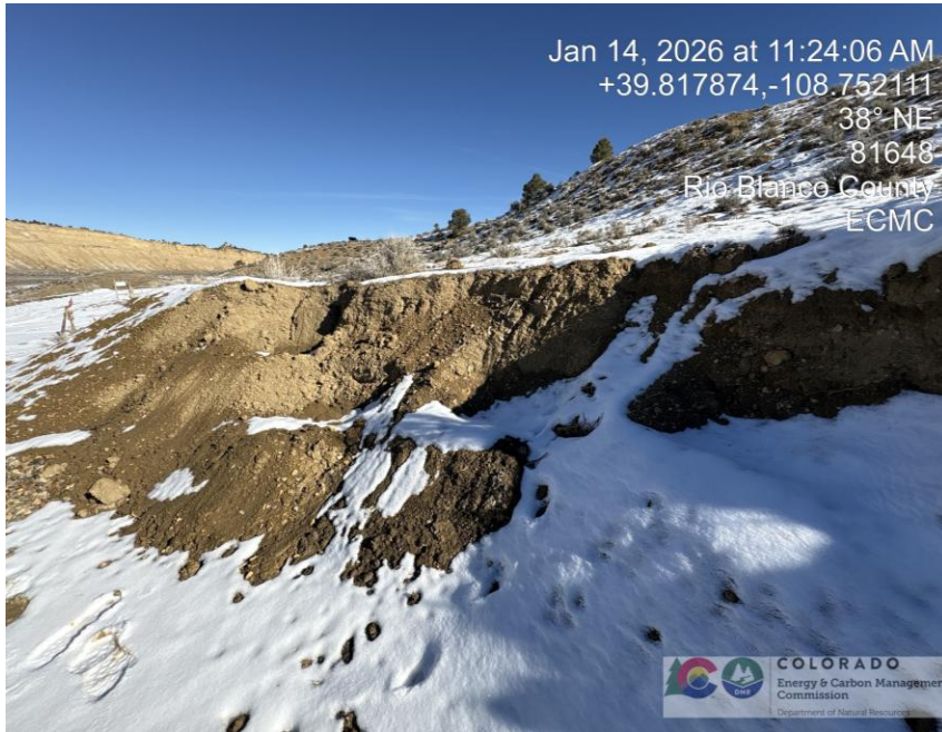
Photo # 1008 Erosion & transport of sediment on cut slope, sediment is migrating onto location near tank battery, the cut slope has experienced progressive erosion and is now actively sloughing, resulting in slope instability.
