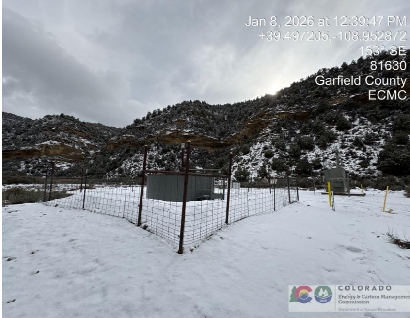
Photo # 0881 NW corner of location
