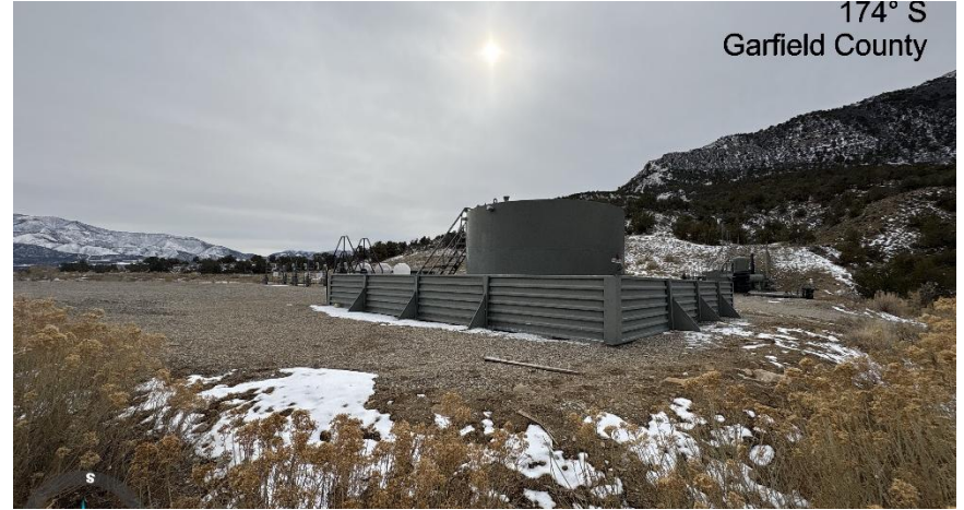
North East corner of location.
