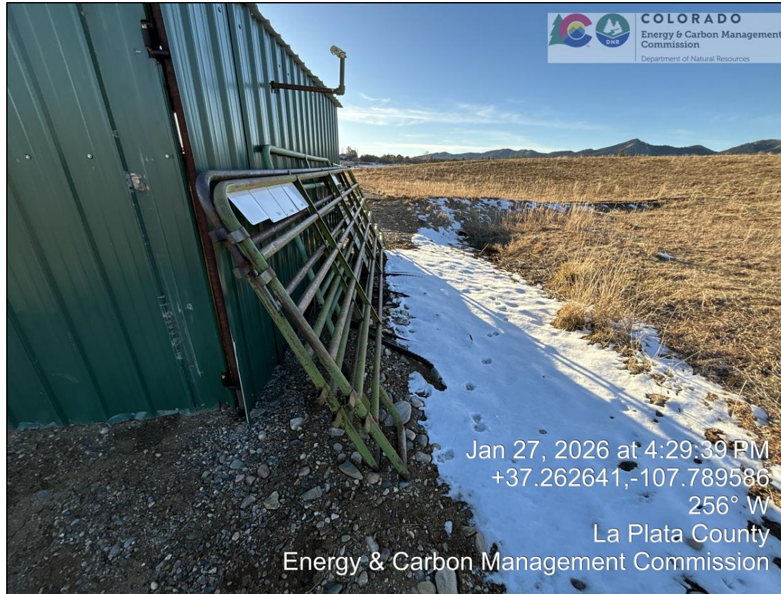
10. Unused hydraulic hose on ground beneath cattle panel fence segments on north side of shed.
