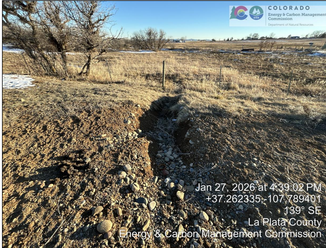
14. Drainage channel where stormwater exits pad.
