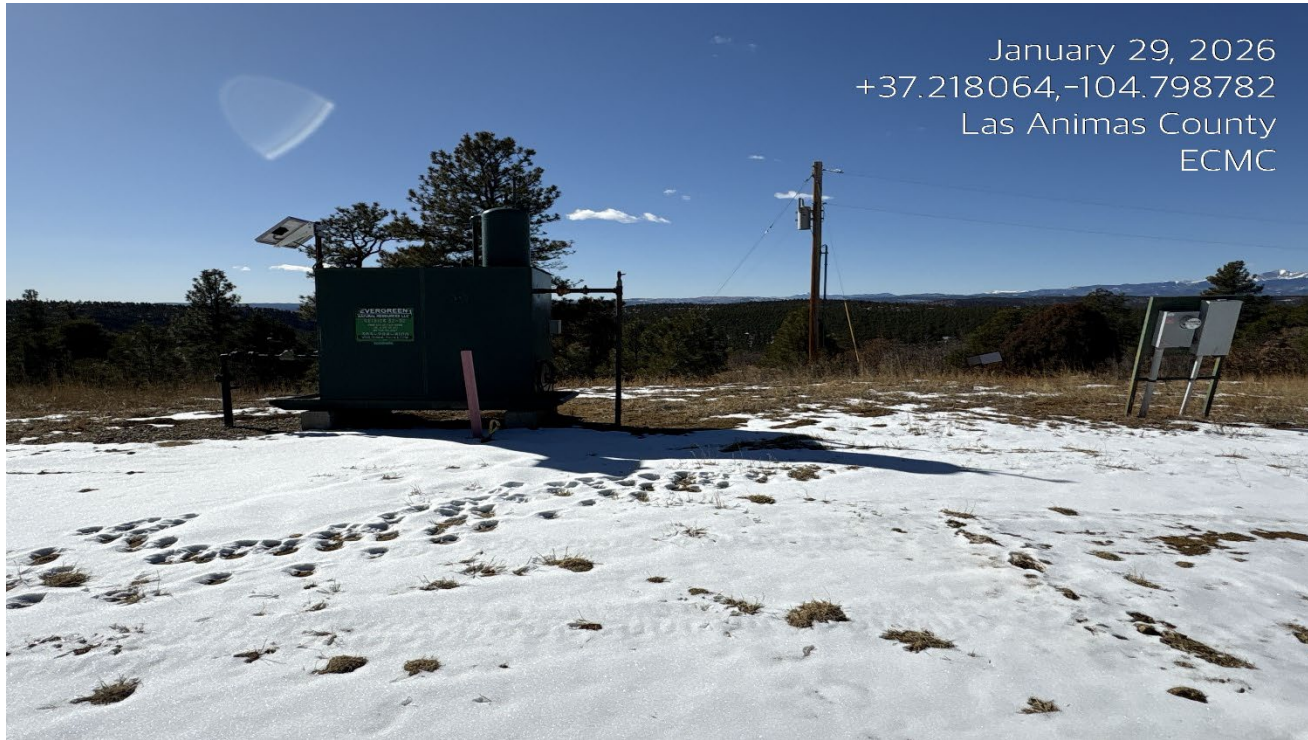
Photo 8. Facing southwest toward the meter shed where the well sign is installed. The wellsite utilizes the electric power line shown in the photo.
