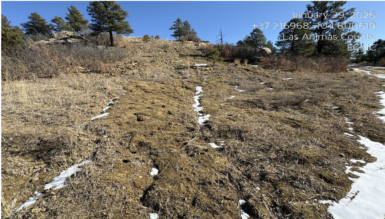
Photo 1. Standing at the access road facing northeast toward the reclaimed flowline ROW. There is erosion along this area that will need to be repaired, reseeded, and stabilized.
