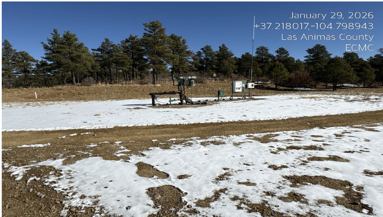
Photo 7. Facing northeast toward the wellsite.
