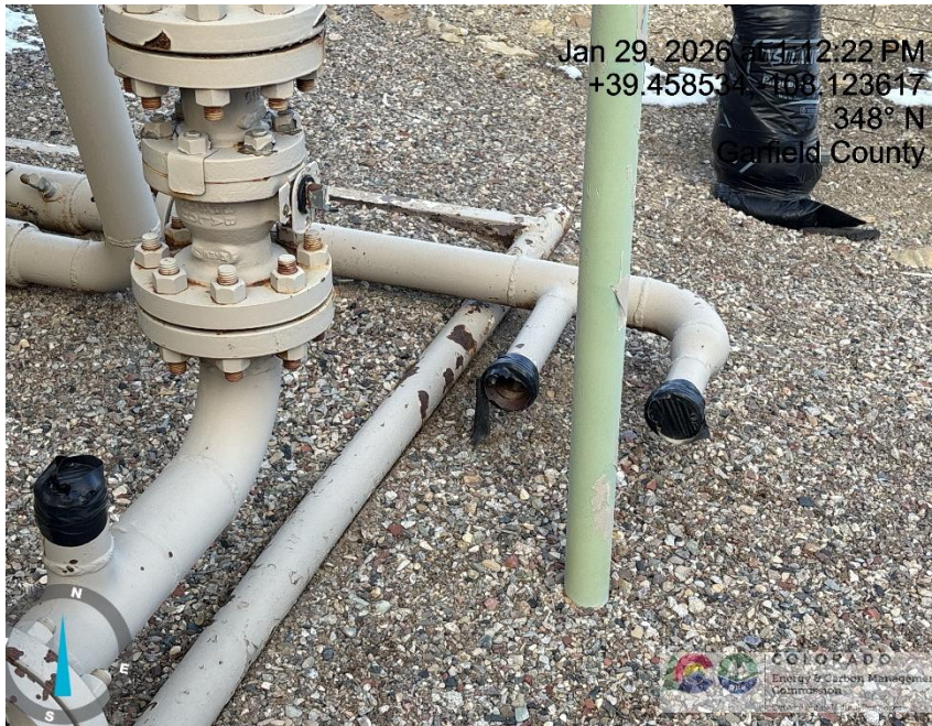
Photo # 7403 Piping on dehy disconnected/dehy not in use/unused equipment – Additionally open ended piping on dehy/wildlife hazard/available for entry by wildlife
