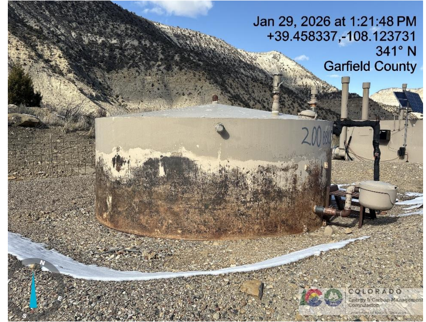
Photo # 7406 Paint peeling off production tank & tank starting to rust
