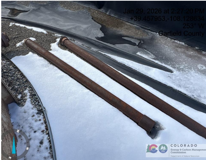
Photo # 7688 Debris in tank battery secondary containment
