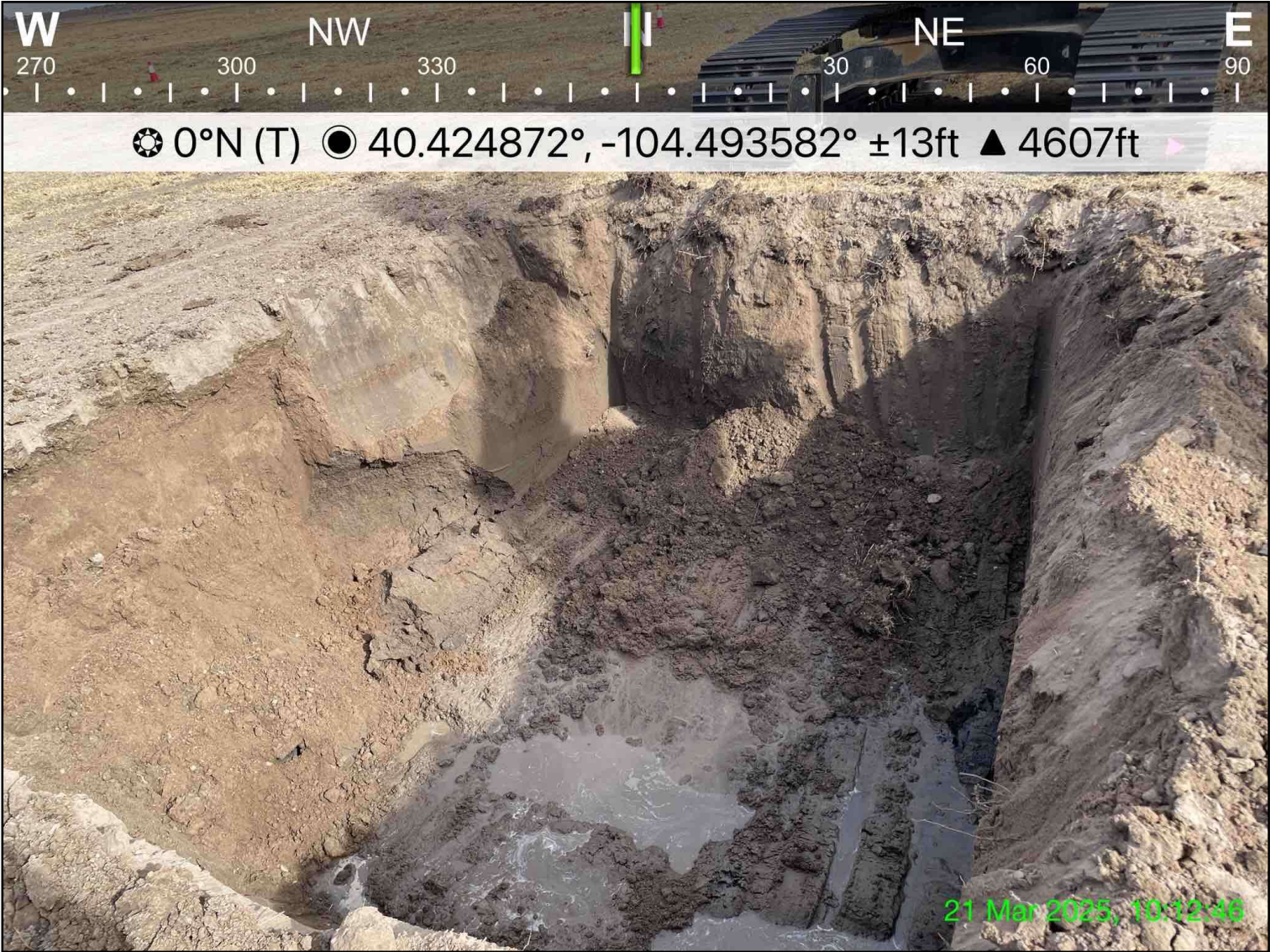
Photo 1: View of wellhead excavation with groundwater infiltration, facing north
