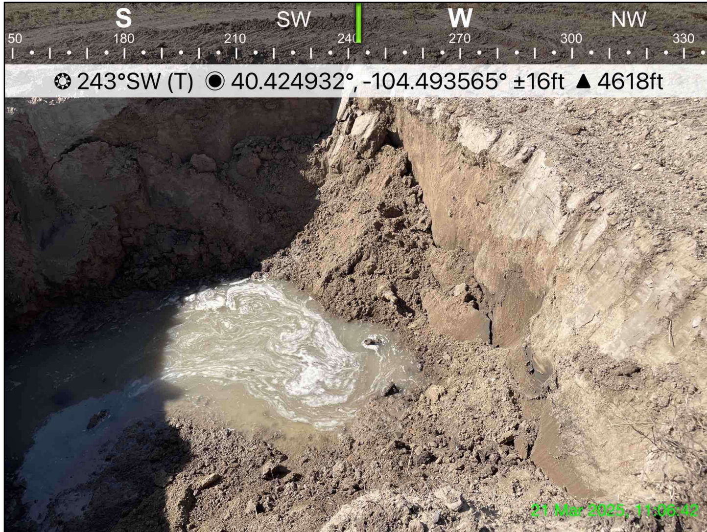
Photo 4: View of wellhead excavation with groundwater, facing southwest
