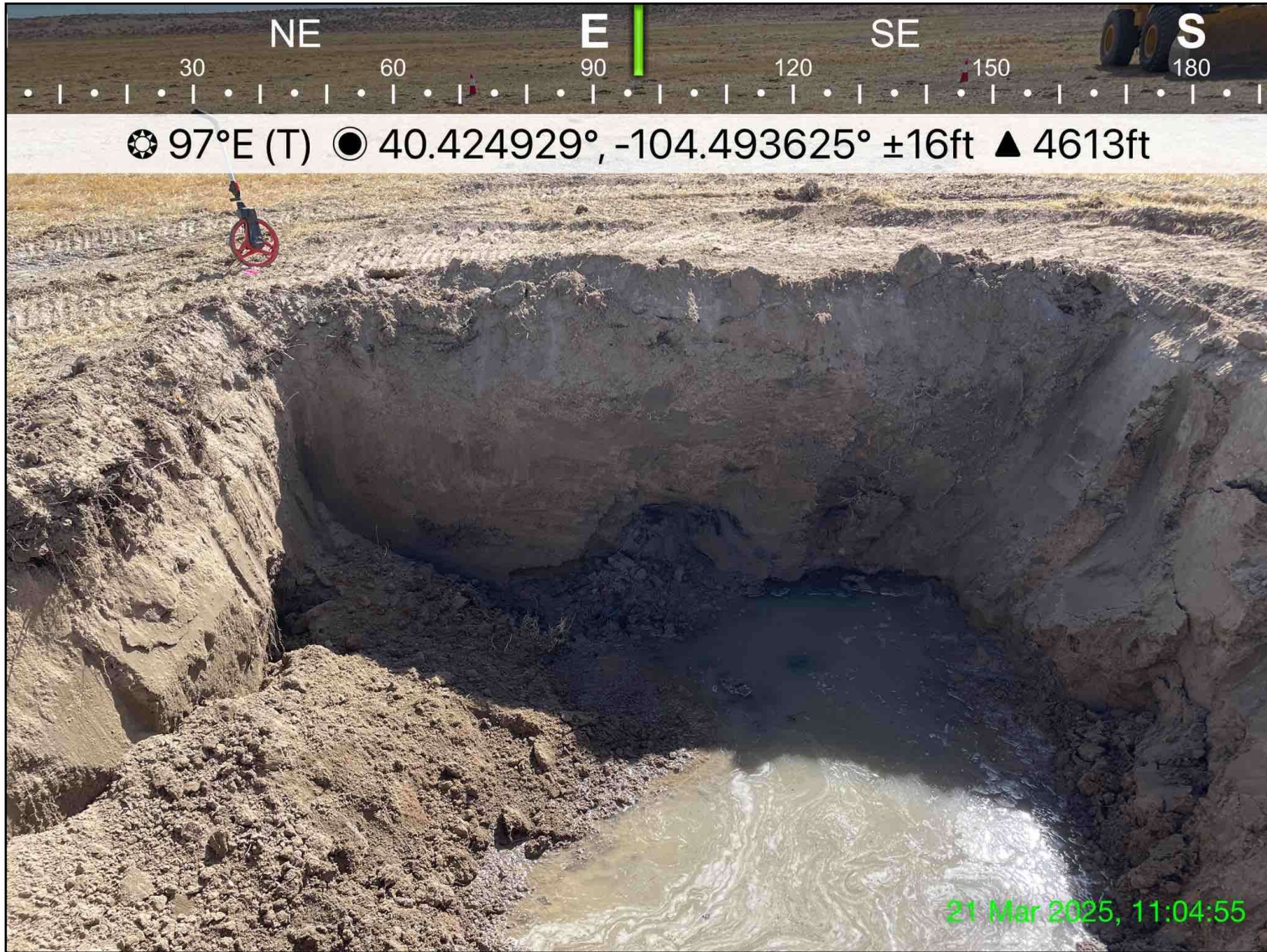
Photo 2: View of wellhead excavation with groundwater, facing east
