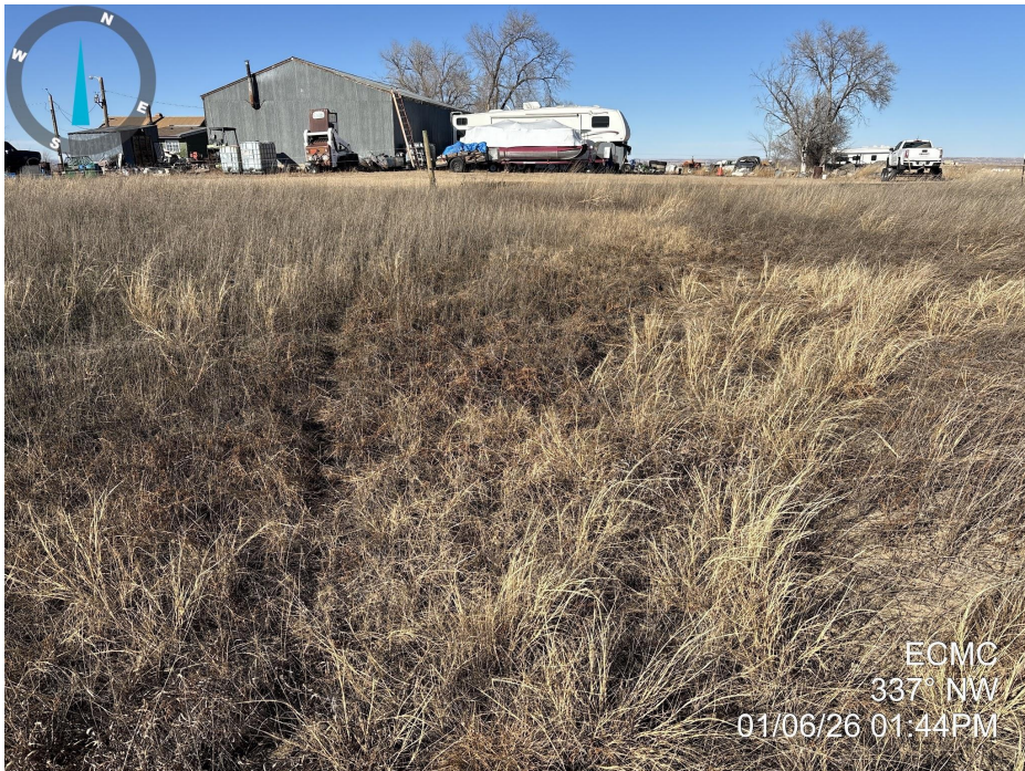
Photo 7. Photo taken of the tank battery location, facing northwest. See comments under Photo 5.
