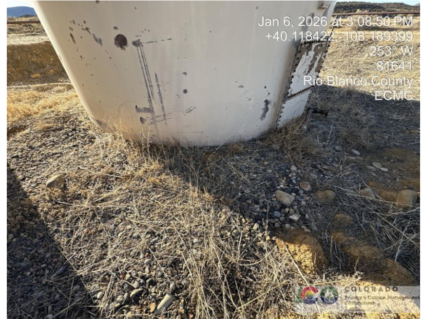
Photo # 0784 Weeds & weed debris in secondary containment presents a potential fire hazard
