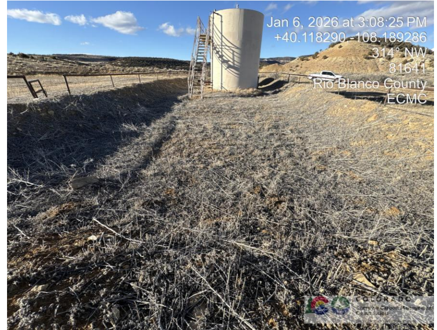
Photo # 0779 Weeds & weed debris in secondary containment presents a potential fire hazard
