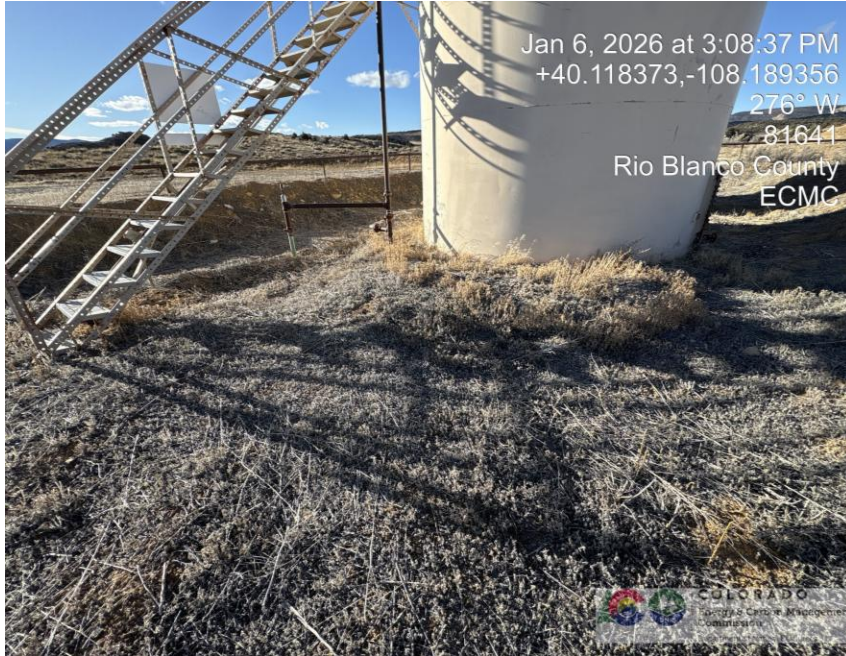
Photo # 0781 Weeds & weed debris in secondary containment presents a potential fire hazard
