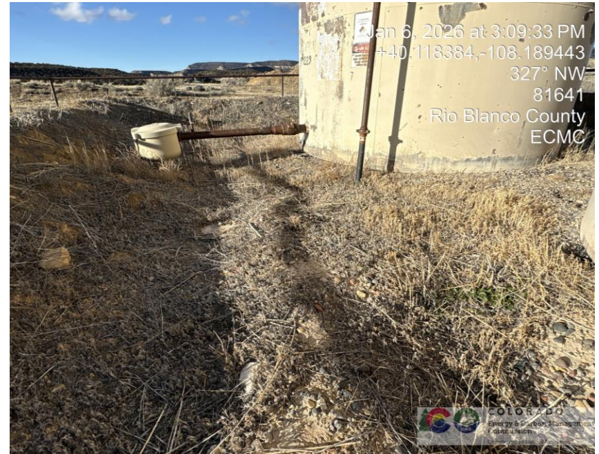
Photo # 0787 Weeds & weed debris in secondary containment presents a potential fire hazard
