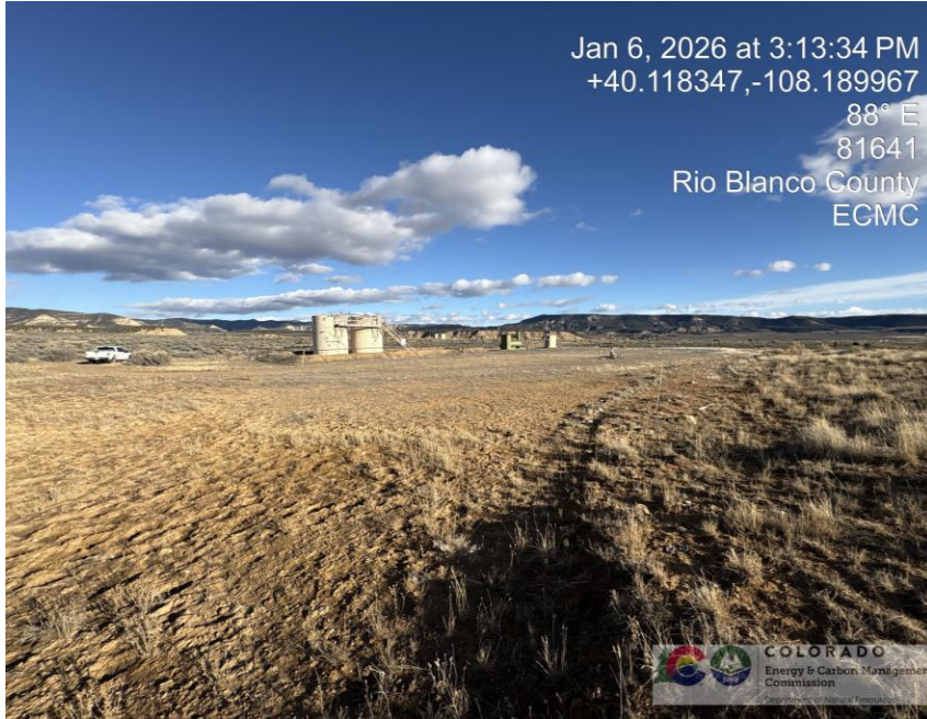
Photo # 0794 NE corner of location
