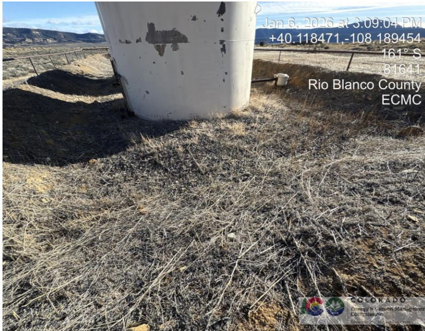
Photo # 0785 Weeds & weed debris in secondary containment presents a potential fire hazard
