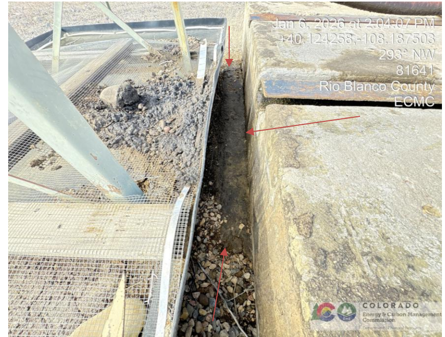
Photo # 0706 Staining on location around Pump Jack
