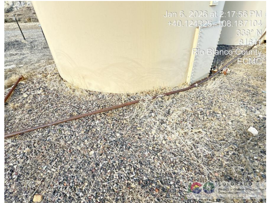
Photo # 0733 Weeds & weed debris in secondary containment presents a potential fire hazard
