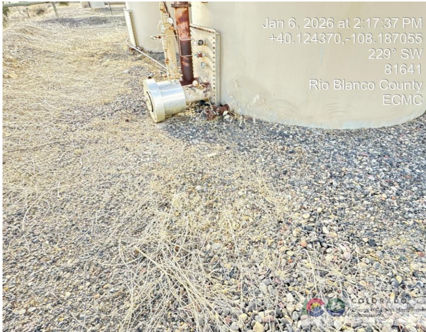
Photo # 0732 Weeds & weed debris in secondary containment presents a potential fire hazard
