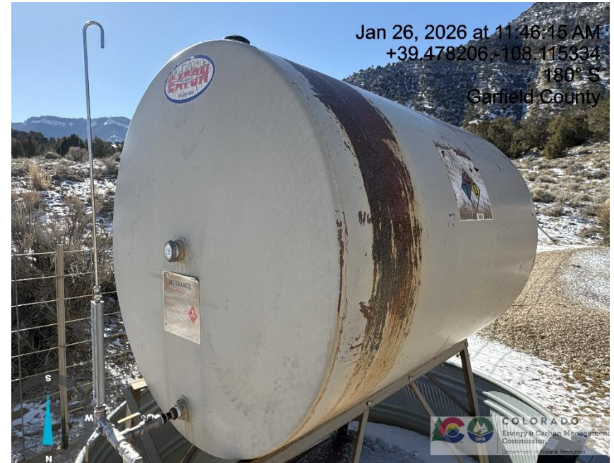
Photo # 4729 Methanol tank label damaged & illegible
