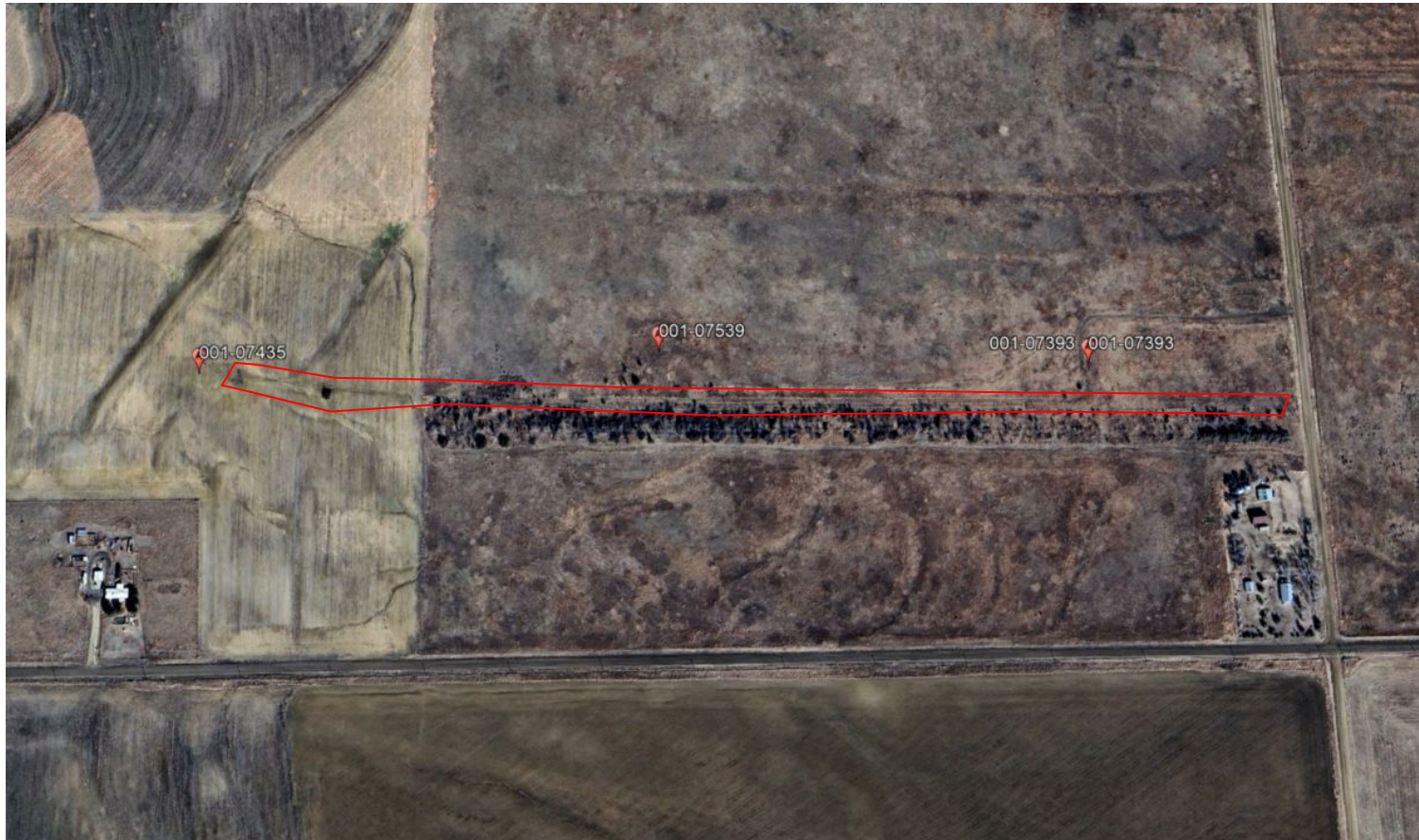
Photo 8. This section of power line appears to have been installed for oil and gas and does not extend past well 001-07435.
