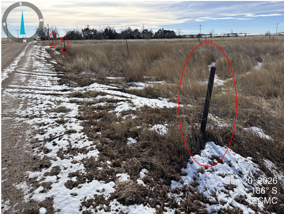
Photo 1. Picture taken on wolf creek rd looking south. Three oilfield pipes are present near the entrances to the tank battery (red circles).
