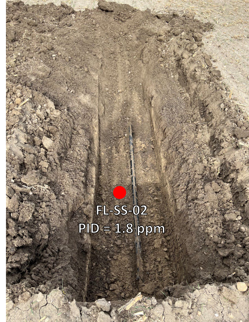
Looking north at bellhole/cut point for removal
